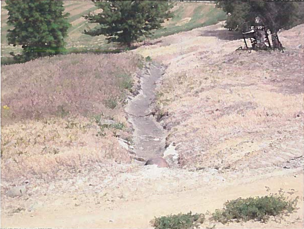
Main drain that delivers water to the 4 acres as shown on the system diagram map. Drain 2 captures the water and conveys the water through the pipe in the picture.
