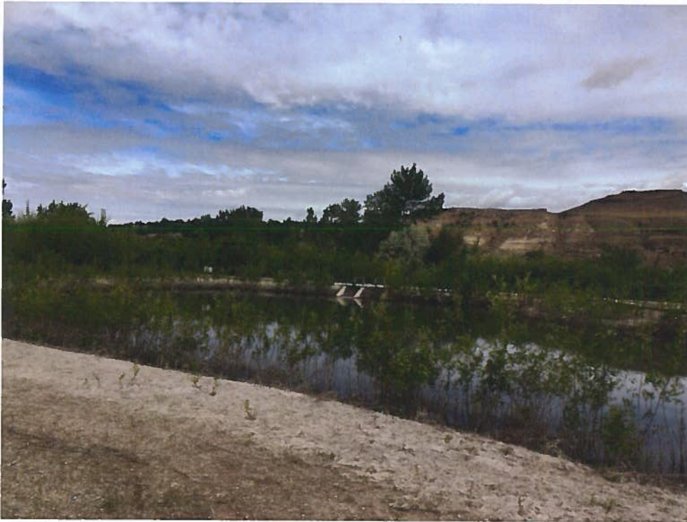
Settling pond looking northwest; note headgate to Williams Pond in background.
