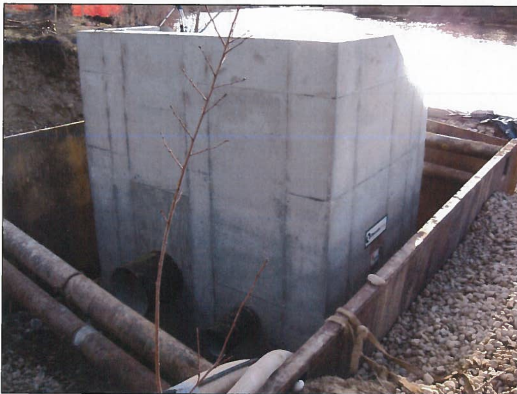
Boise River diversion structure during installation in 2010
