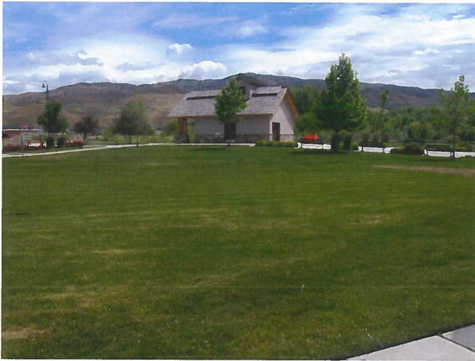
Pump house building with pressurized irrigation pumps and wet well
