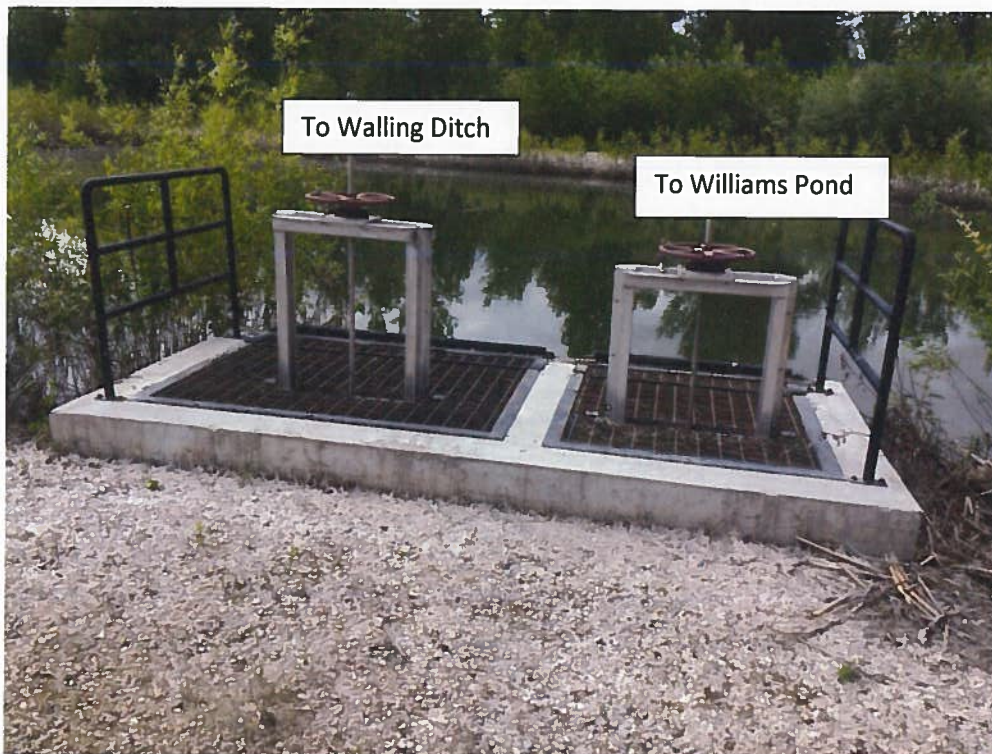
Headgates on settling pond
