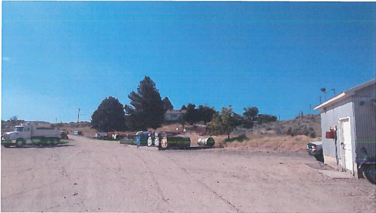
Figure 3 Looking south towards the home where water is used for domestic purposes from the pumphouse
