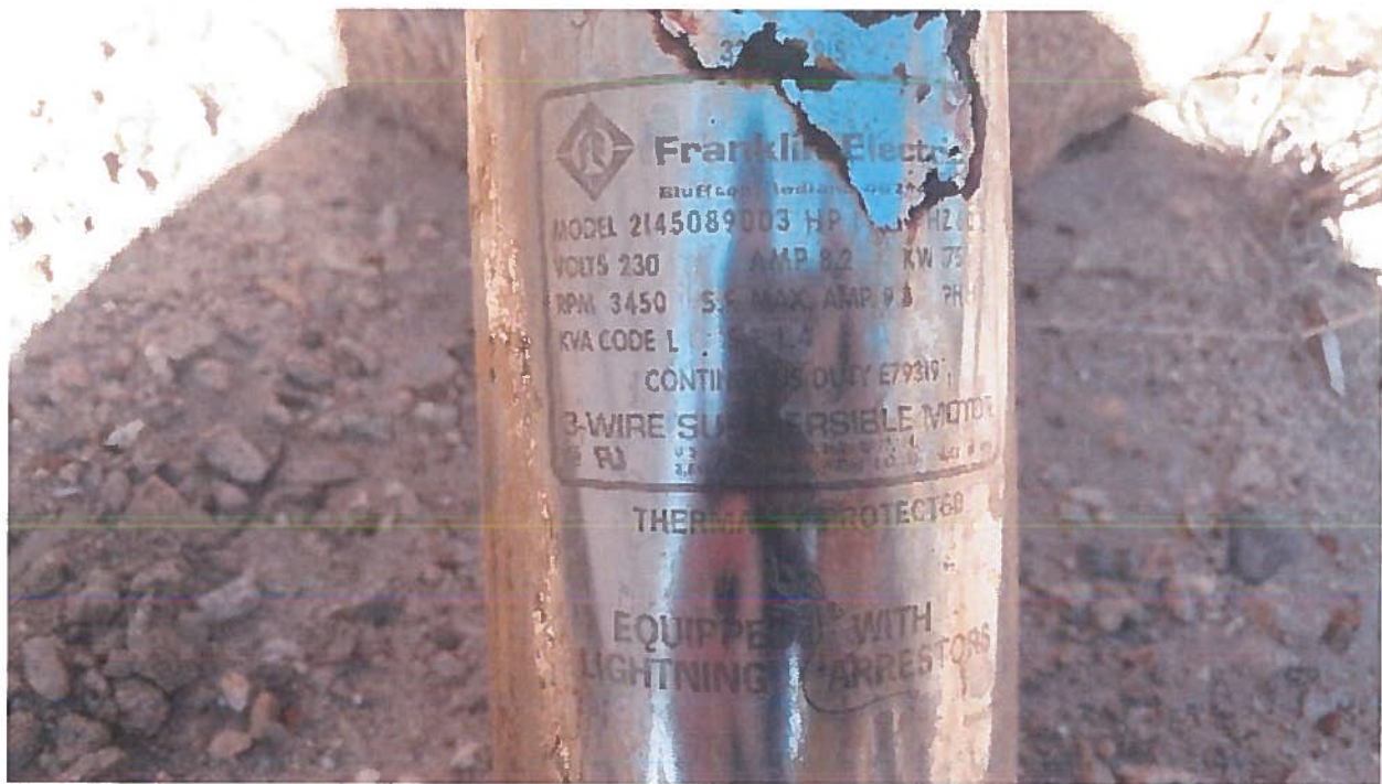
Figure 1 The 1-hp pump that was replaced shortly before the site visit. Parameters such as dynamic WL and mainline pressure remain unknown making estimation of flow rate difficult.
