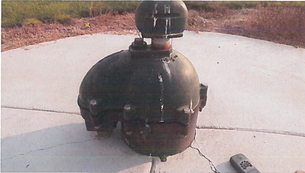
Figure 1 The well head for the POD. There is currently no metal tag welded to the casing, but a well log matching the dimensions of the well give a tag no. of D0057615.
