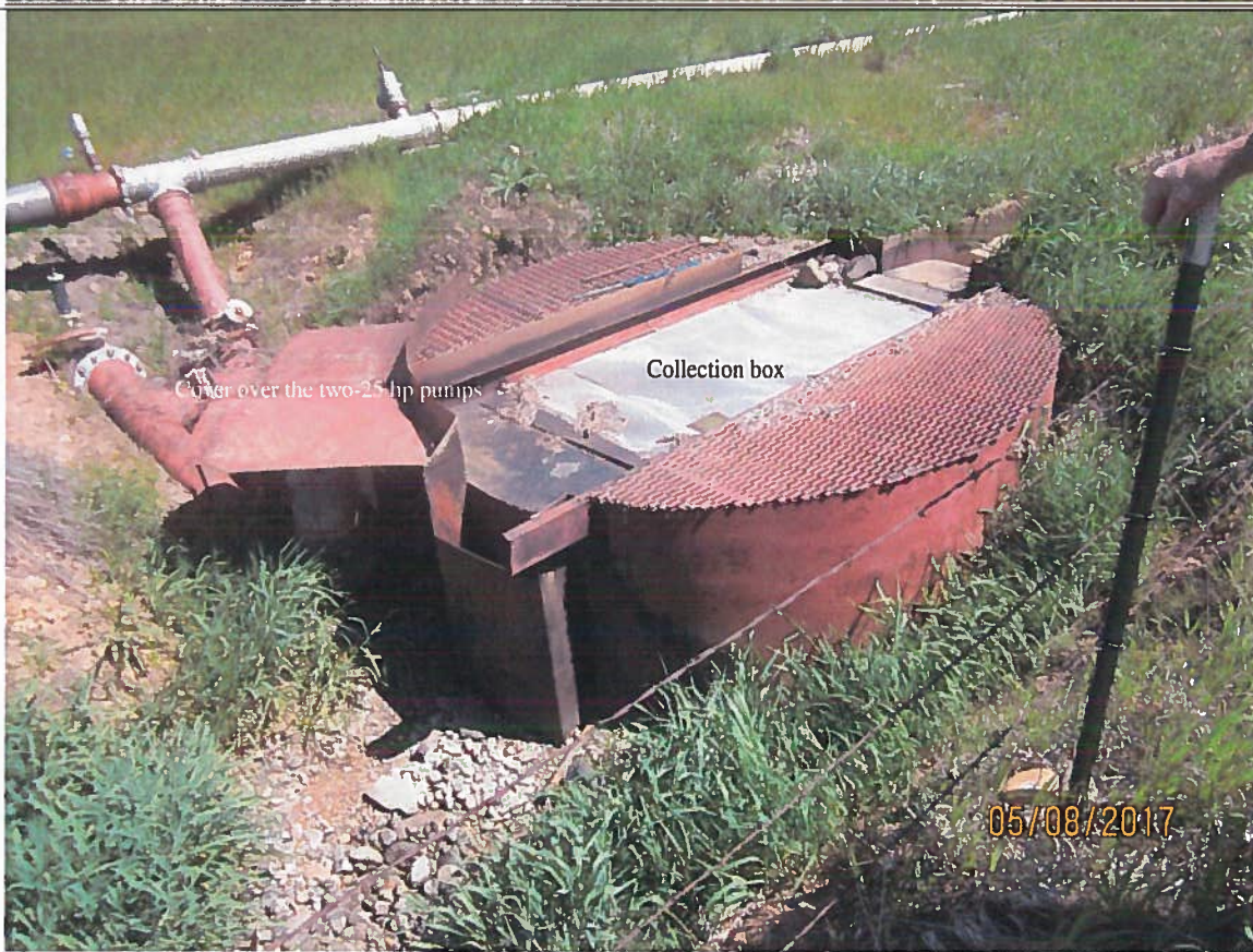
Collection box along Gray's Creek Road. Two-25 hp pumps divert the water through an 10" steel pipe to the pivots.
