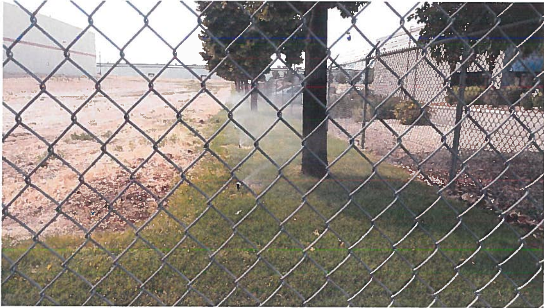
Figure 7 Pop-up sprinklers at the western edge of the property. The flow rate for pop-up is estimated at ~ 3gpm.
