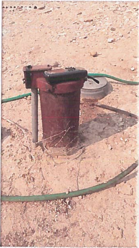
Figure 1 The well head located in the NESW of Sec 9 T03N R01E B.M. There is no record of this well in the IDWR database nor is there a metal tag welded to the casing. The well was apparently constructed in 1968.
