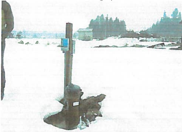
Photograph 5: Well #2 looking toward pump house
