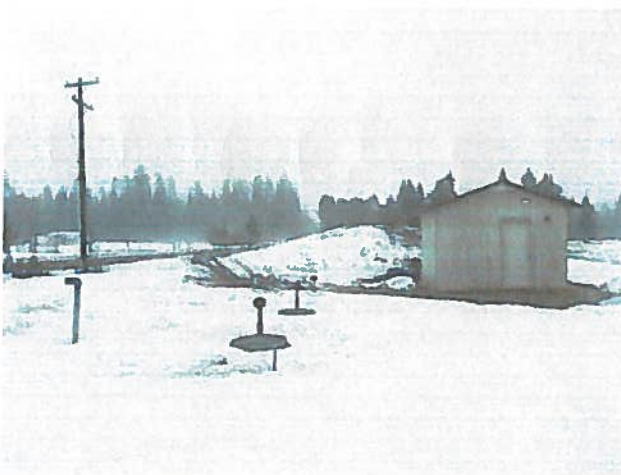
Photograph 21: Fire storage tanks and pump house
