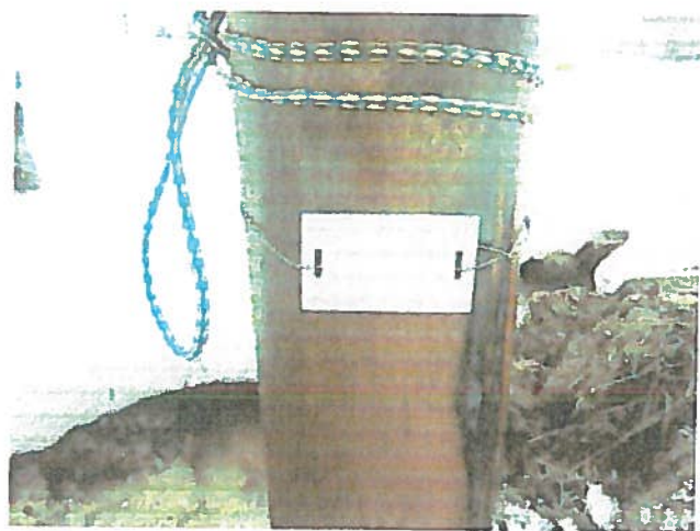
Photograph 4: Well #2 (DEQ well tag# E0010051)
