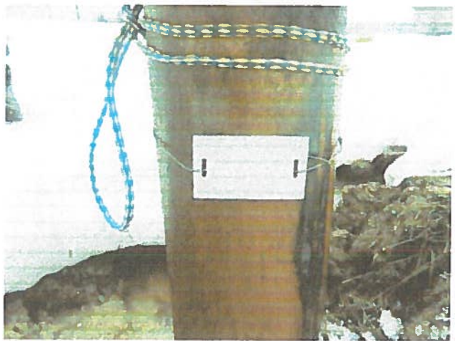
Photograph 4: Well #2 (DEQ well tag# E0010051)
