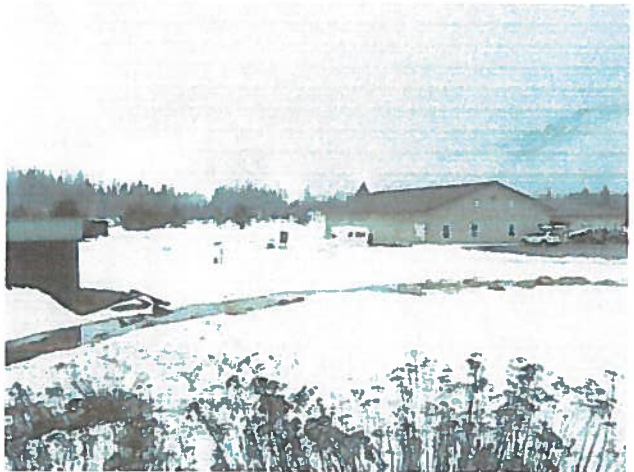
Photograph 20: Looking toward church from storage tanks
