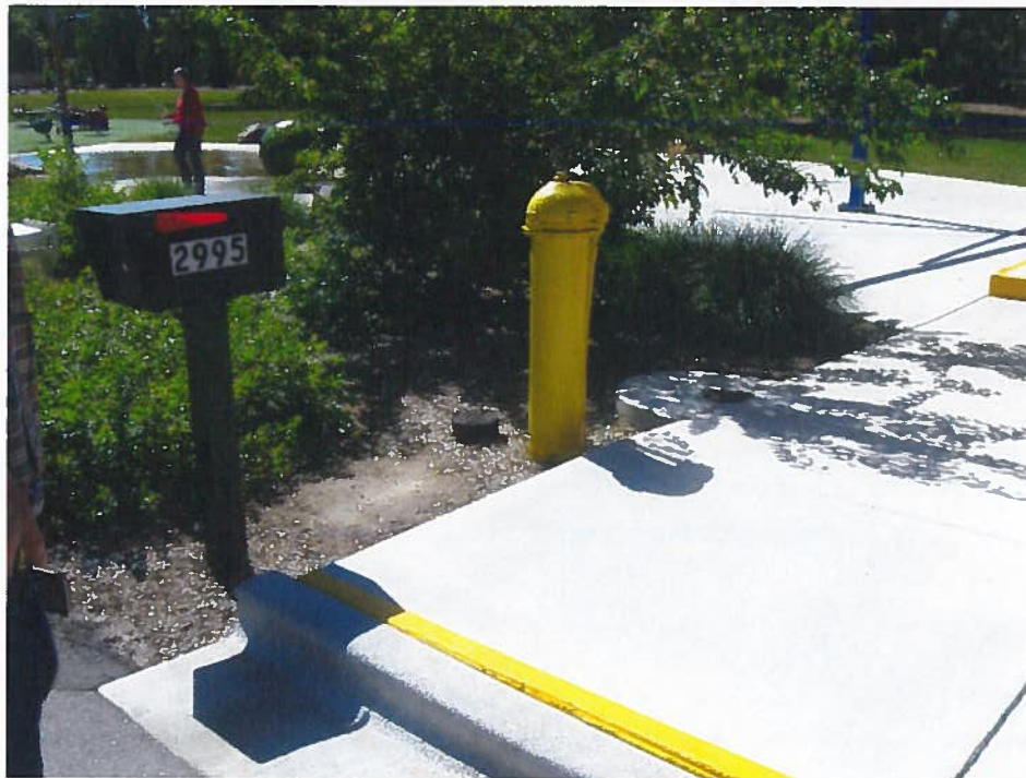
Wet well location for spray-park reuse pump
