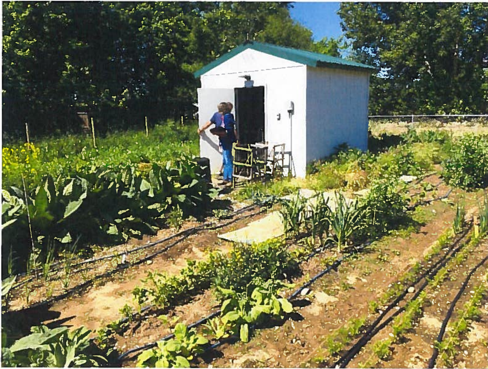
Ground water and surface water pump house
