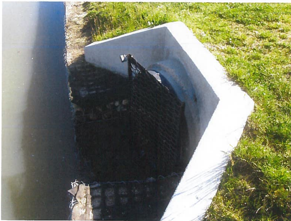
Surface water inlet on east side of pond 2
