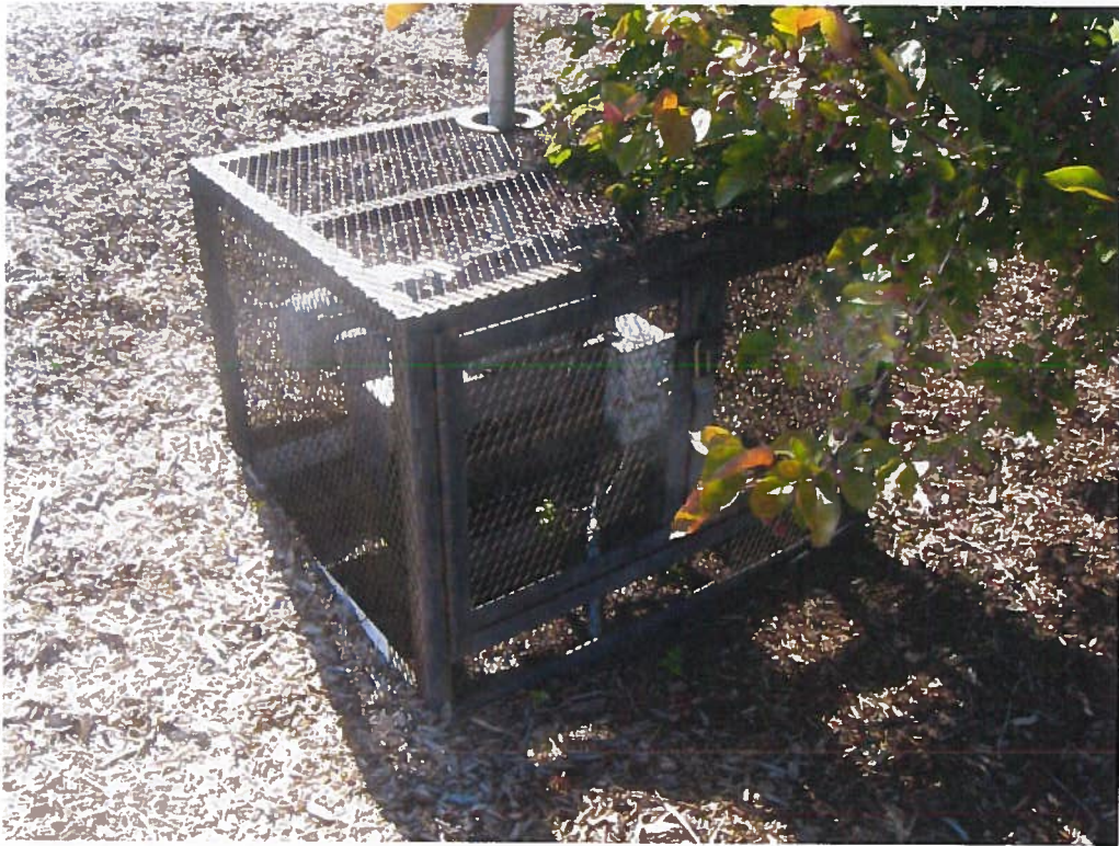
Surface water automatic headgate to pond 2
