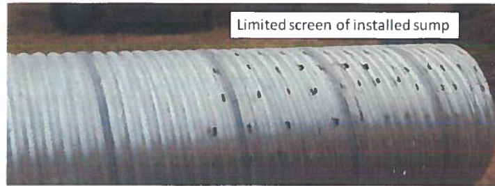
Figure 4: CMP installed showing limited perforations for screen.
