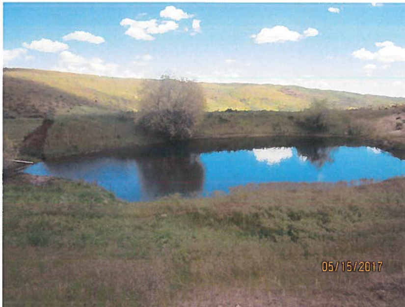
Figure 2 The pond known as West 2. The washed-out dam can be seen in the picture to the left.
