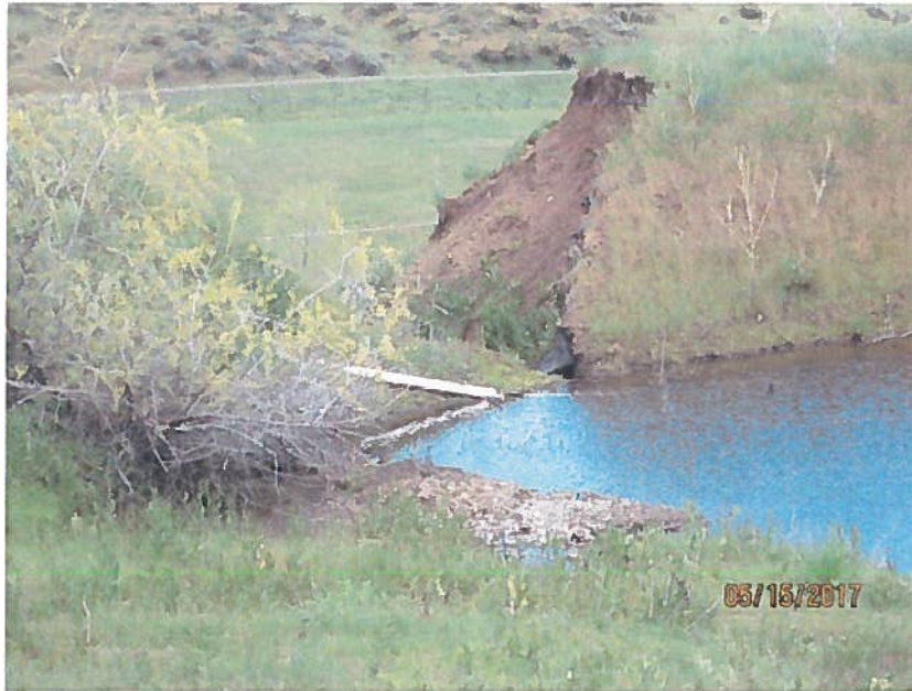
Figure 3 A closer look at the washed-out dam for West 2.
