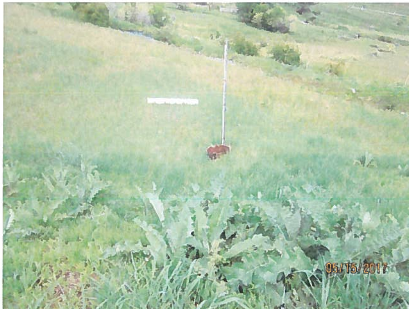
Figure 4 Another valve, this at the foot of the dam for West 2. When open, water from West 2 moves downslope to risers which are tied to the wheel line and used for irrigation.
