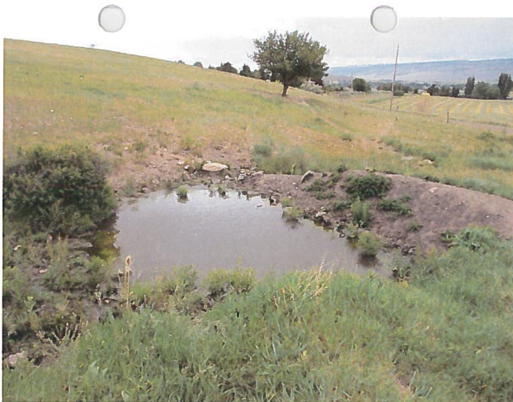
Upstream view of pond, with stream entering pond at lower left, exiting top center.
