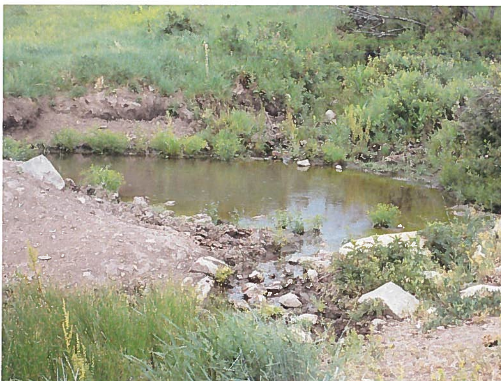
Downstream view of pond. Outlet is at bottom center.
