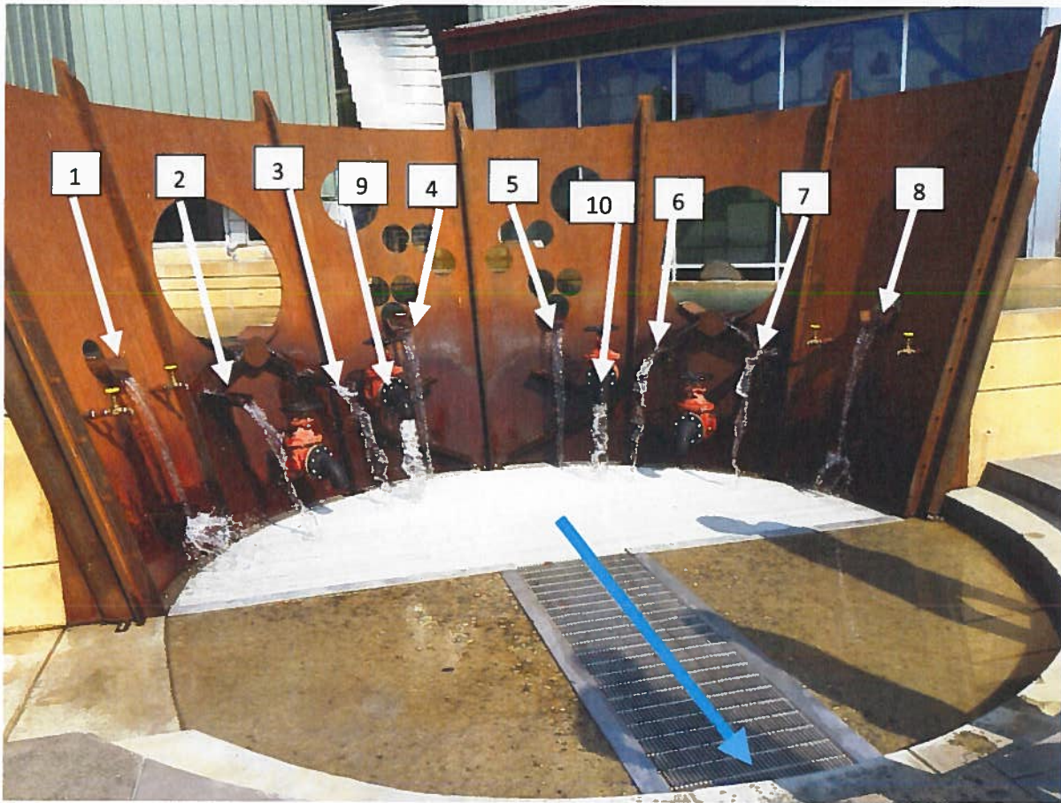
Discharge ports used for timed flow measurements (measurement numbers correspond to table). Well discharges to storage reservoir and base of fountain through 6-inch buried pipeline. All water overflows from reservoir at this point to a drain. Drain channel flows beneath stainless steel grates and concrete walk and discharges to the simulated stream.
