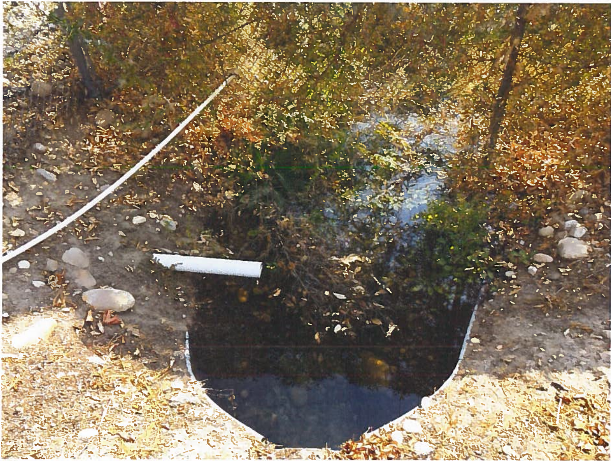
Open waste ditch east of Ancell Avenue for infiltration/conveyance of wastewater from exhibit
