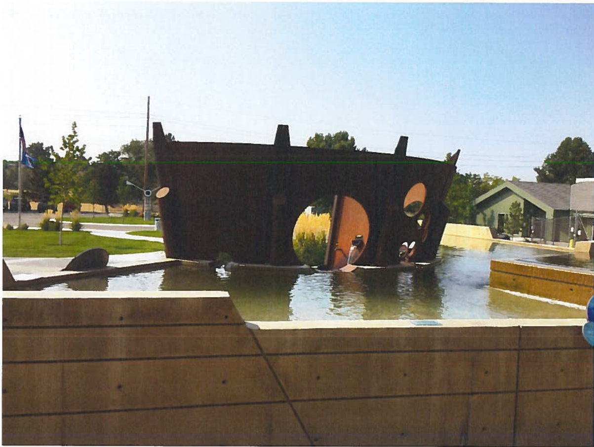
Reservoir looking toward overflow
