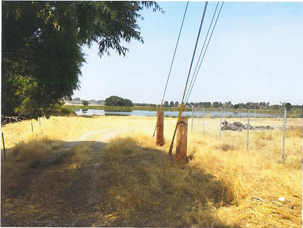
Pond west of wastewater treatment plant. Wastewater from Boise Watershed Exhibit can potentially be discharged to this pond; however, all water was infiltrating before reaching pond at time of exam
