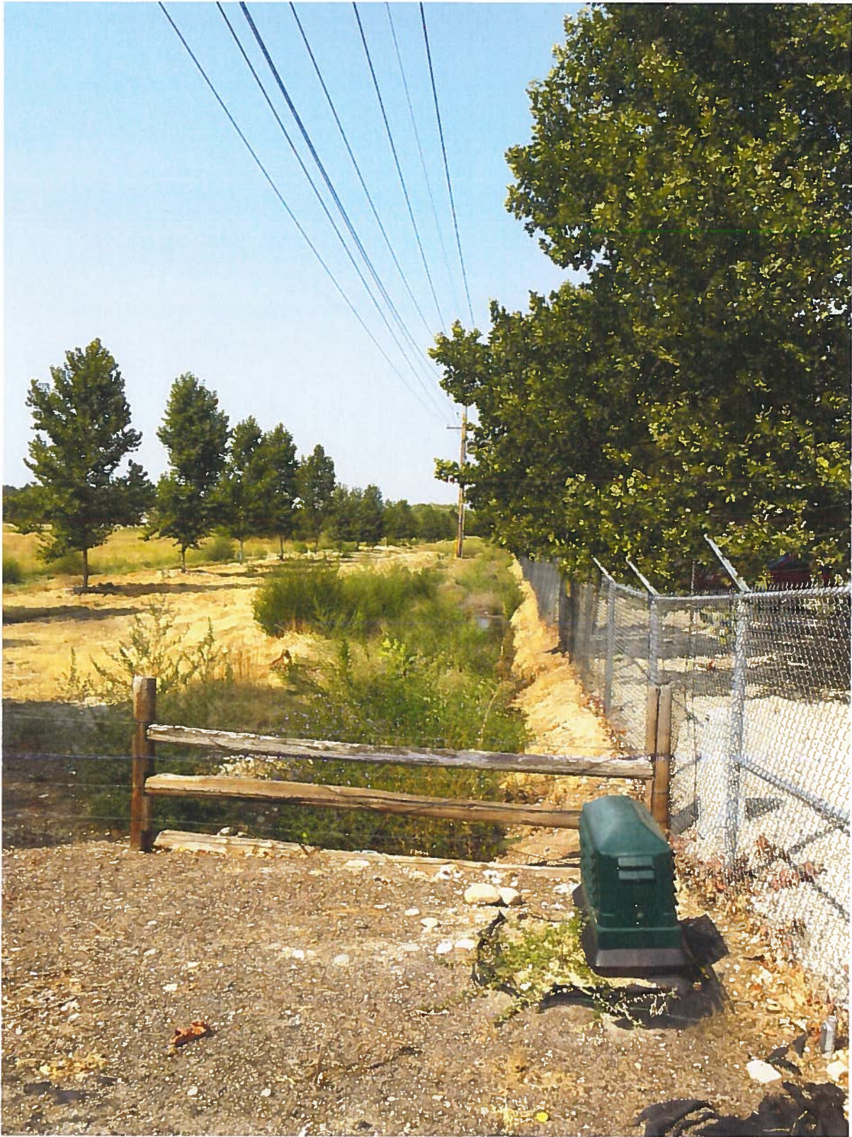
Open waste ditch west of Ancell Avenue for infiltration/conveyance of wastewater from exhibit
