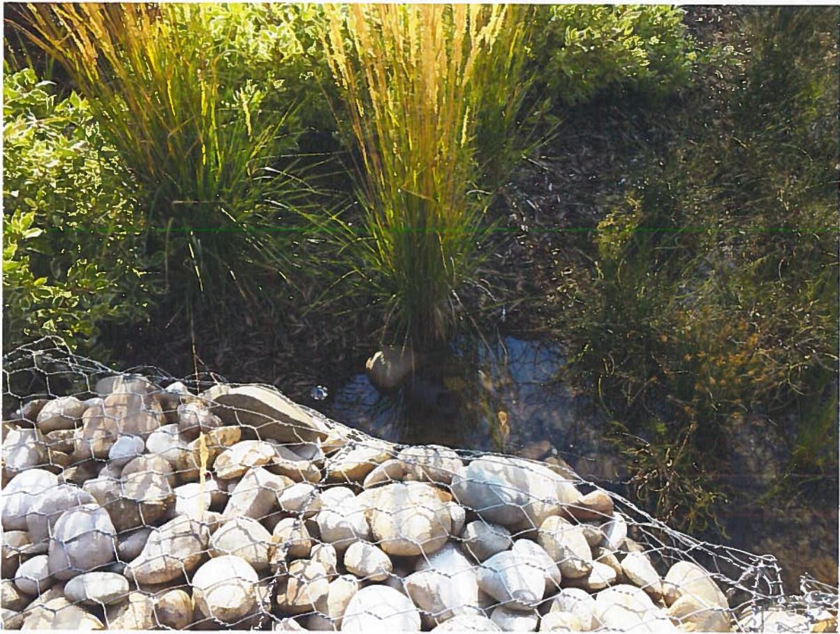
Discharge pipe to wetlands
