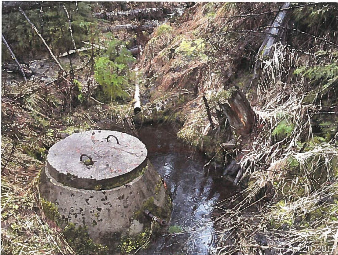
Photo 4 (April 20 2017) – Basin once used for drinking water for abandoned adjacent property; no connection found to empty Pond in Photo 6.
