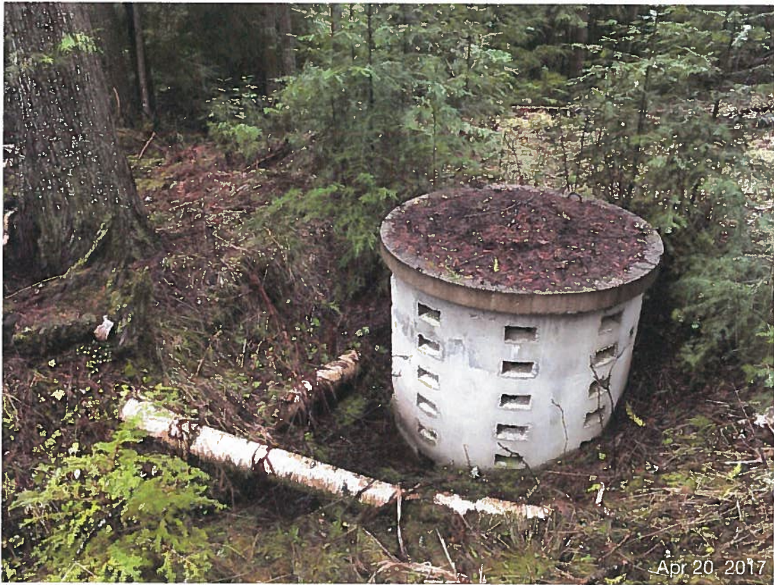
Photo 5 (April 20 2017) – Reportedly abandoned basin; no connection found to empty Pond in Photo 6.
