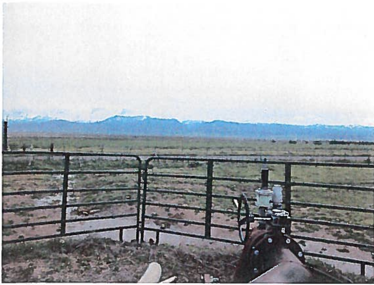
Looking at pipe that is running out to North Pivot
