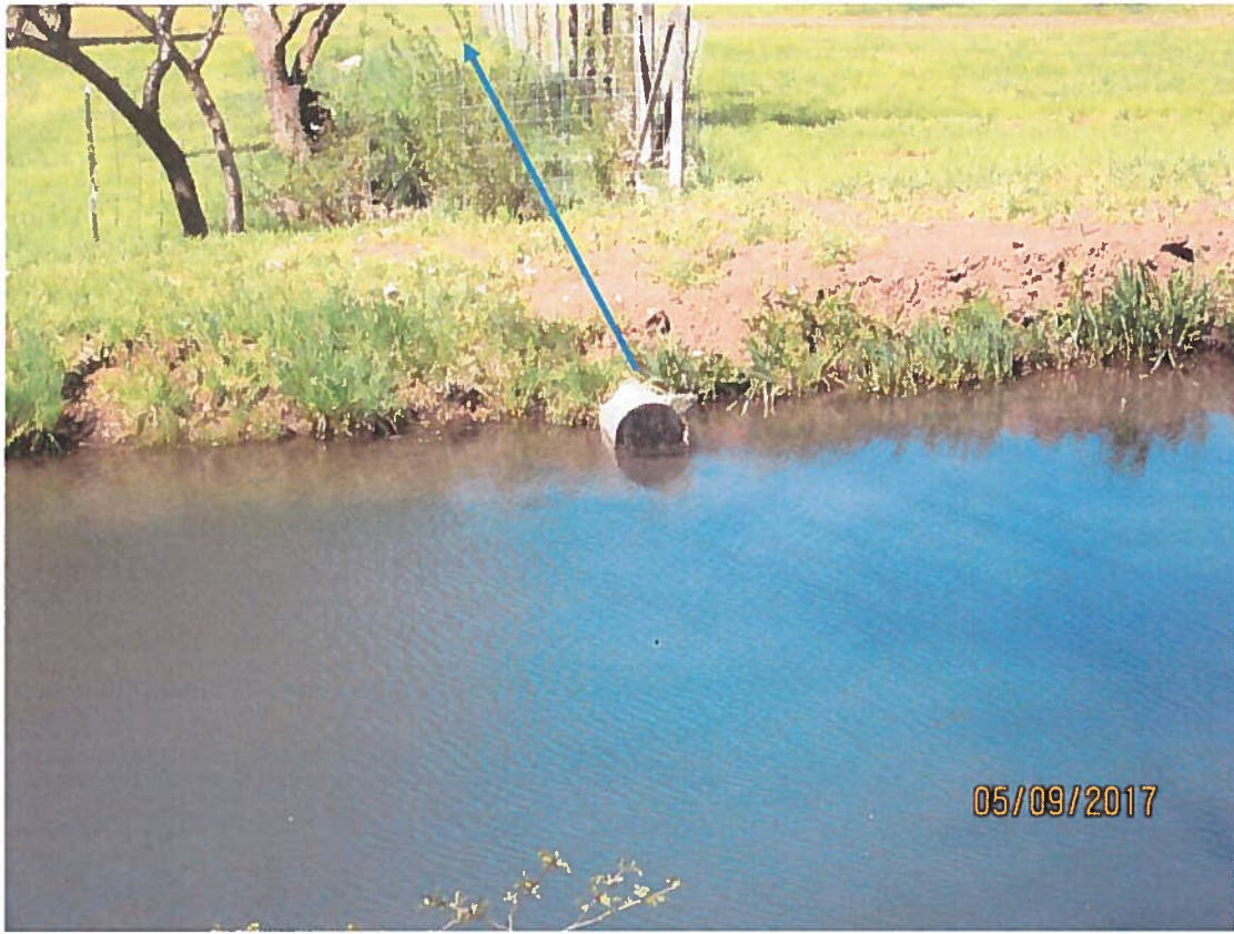
Overflow outlet that conveys water to the west pond and irrigation water around the garden area and house.
