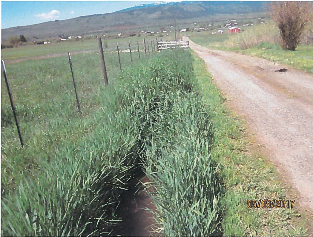
Ditch along the driveway that conveys water to the west pond.
