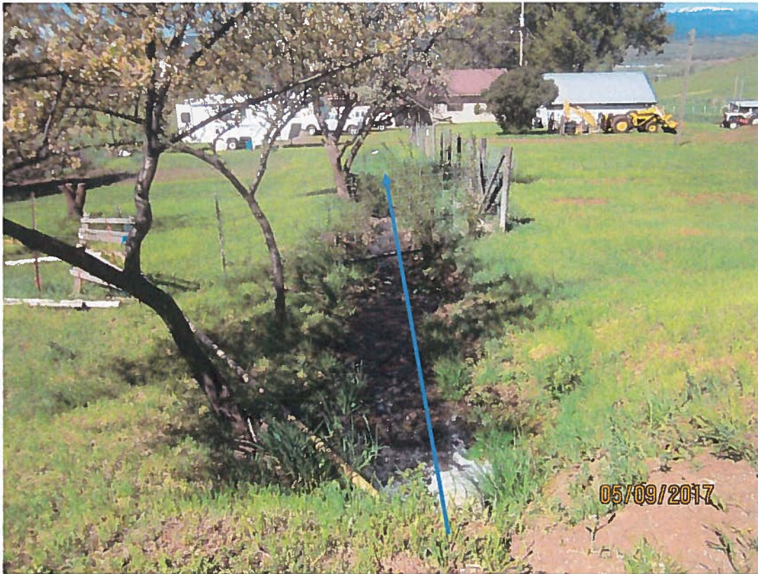
Ditch that conveys water to the west pond.
