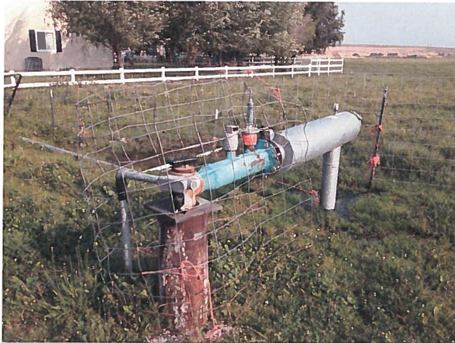
Figure 1 The 294-foot deep, 10-inch diameter irrigation well.
