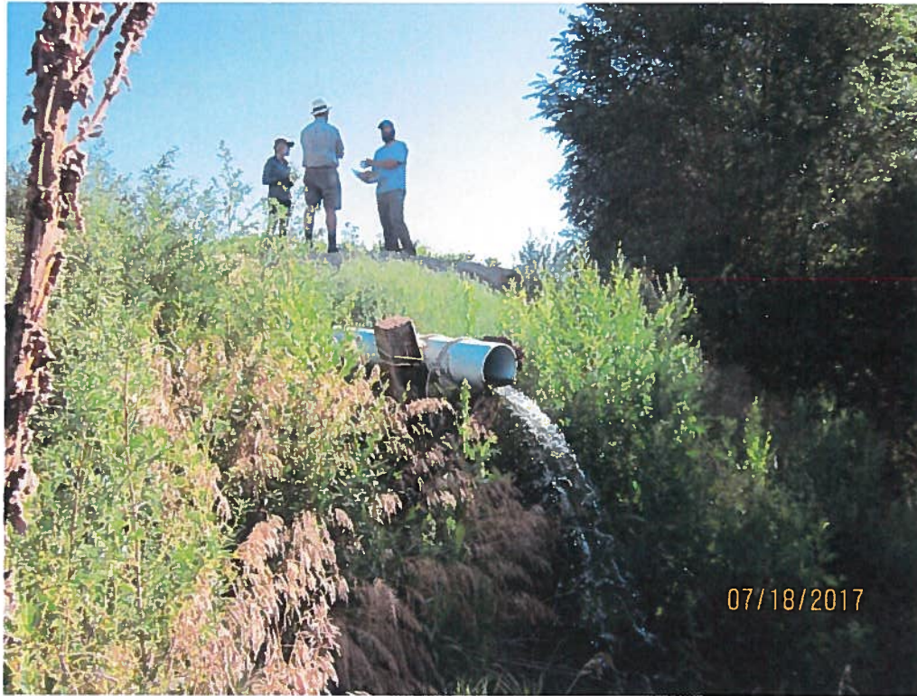
The outlet pipe for the reservoir. There is a second outlet pipe that isn't visible, behind the bushes that serves as an emergency outlet.
