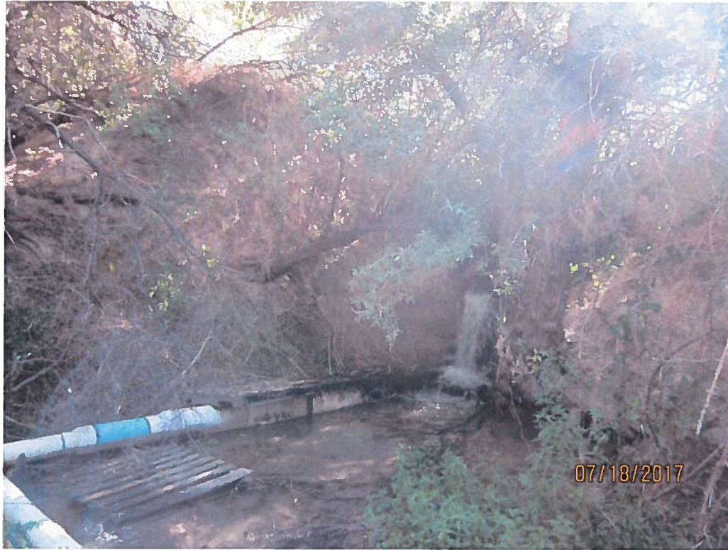
The diversion is created by a PVC pipe positioned vertically in the downpour from the culvert.
