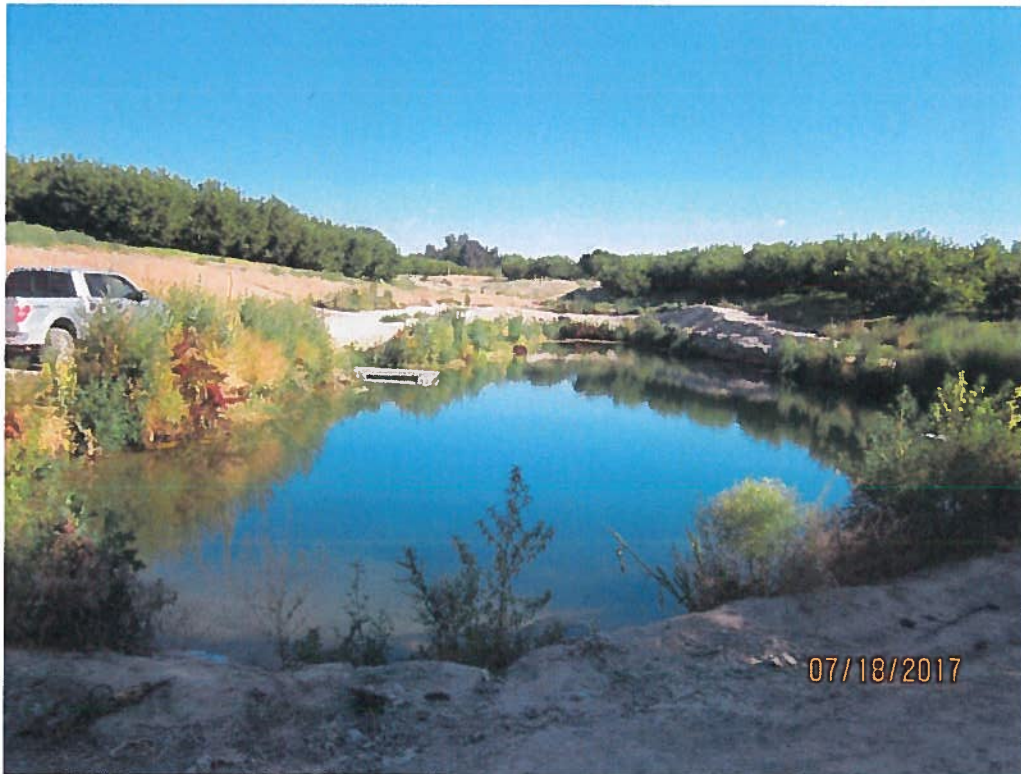
Looking northwest from the embankment across the storage pond. Water from the diversion system enters the pond near the far end of the pond.
