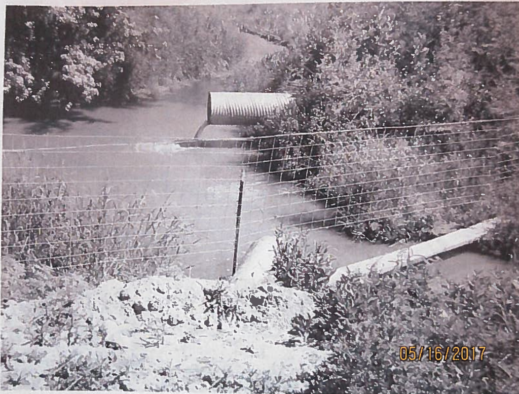
Discharge of the water into the North Drain. Photo received from Mary Trail.
