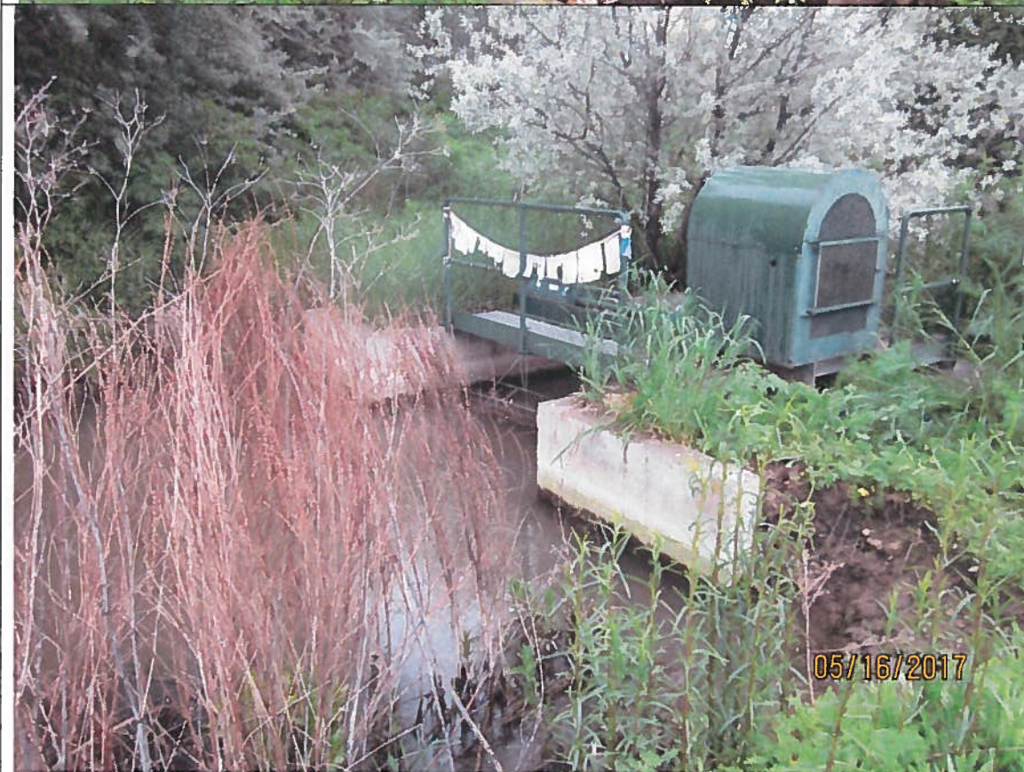
Downstream of the control gate.
