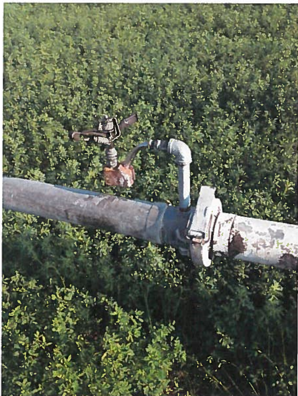
Figure 3 A totalizing flow meter is installed at the diversion but does not appear to be functioning properly.
