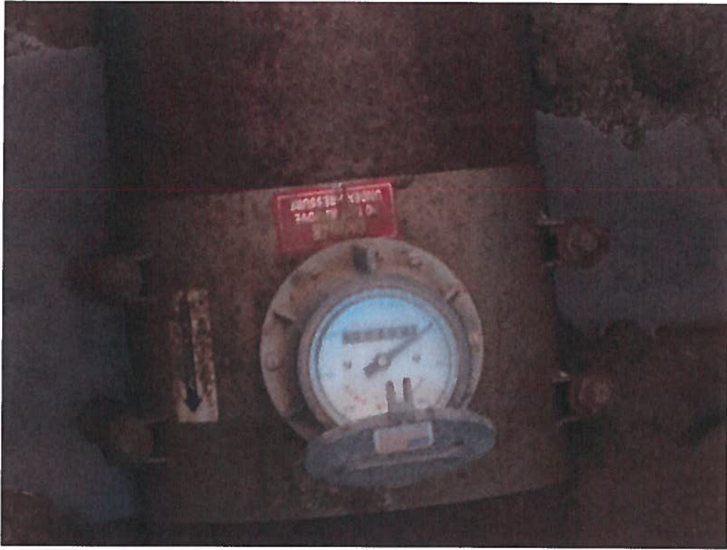
Figure 3 A totalizing flow meter is installed at the diversion but does not appear to be functioning properly.
