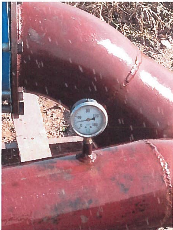
Figure 2 The pressure gauge located at the well head. The gauge did not appear to be functioning properly at the time of the exam.
