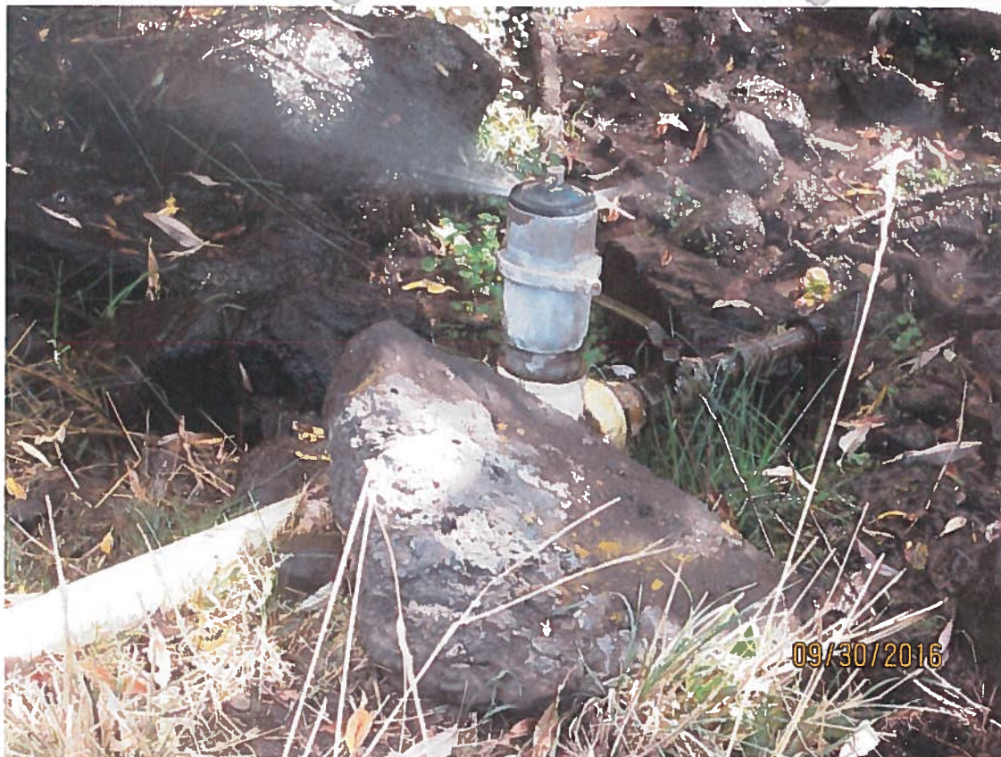
The very last riser in the irrigation system. This riser is found along the creek in the SENW QQ of section 11.
