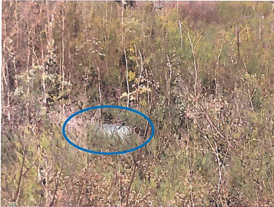
Figure 5 Low-resolution picture of the aluminum culvert from the concrete box leading into the northern flood cell.
