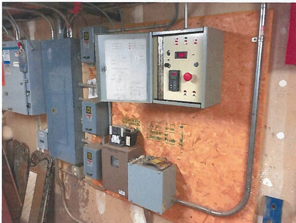
Heating/Cooling System Controlling Works
