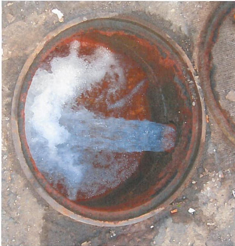
Discharge to storm drain manhole
