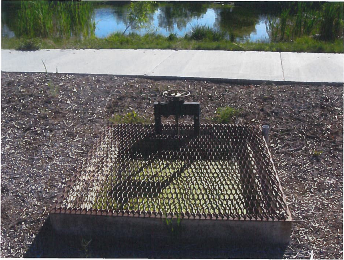
Inlet from irrigation lateral to pond.
