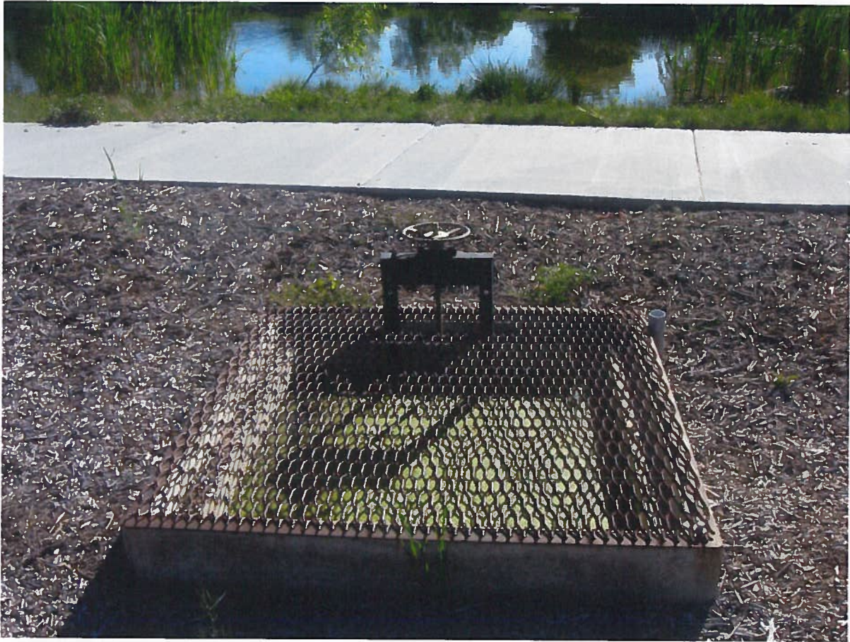
Inlet from irrigation lateral to pond.
