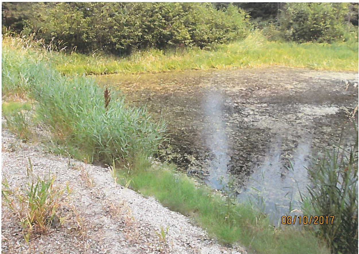
Standing on dam looking north.
