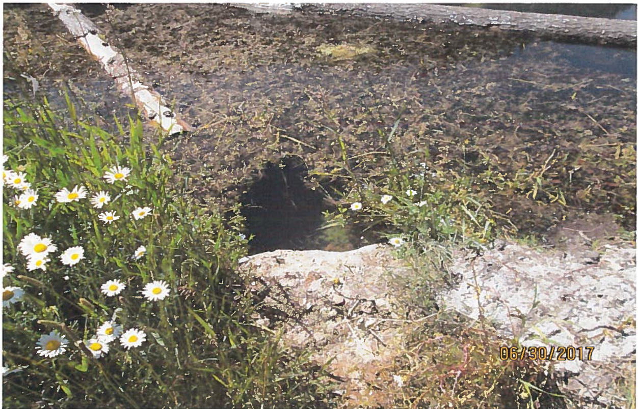
Overflow culvert in between pond 2 & 3. View is looking at pond 3.
