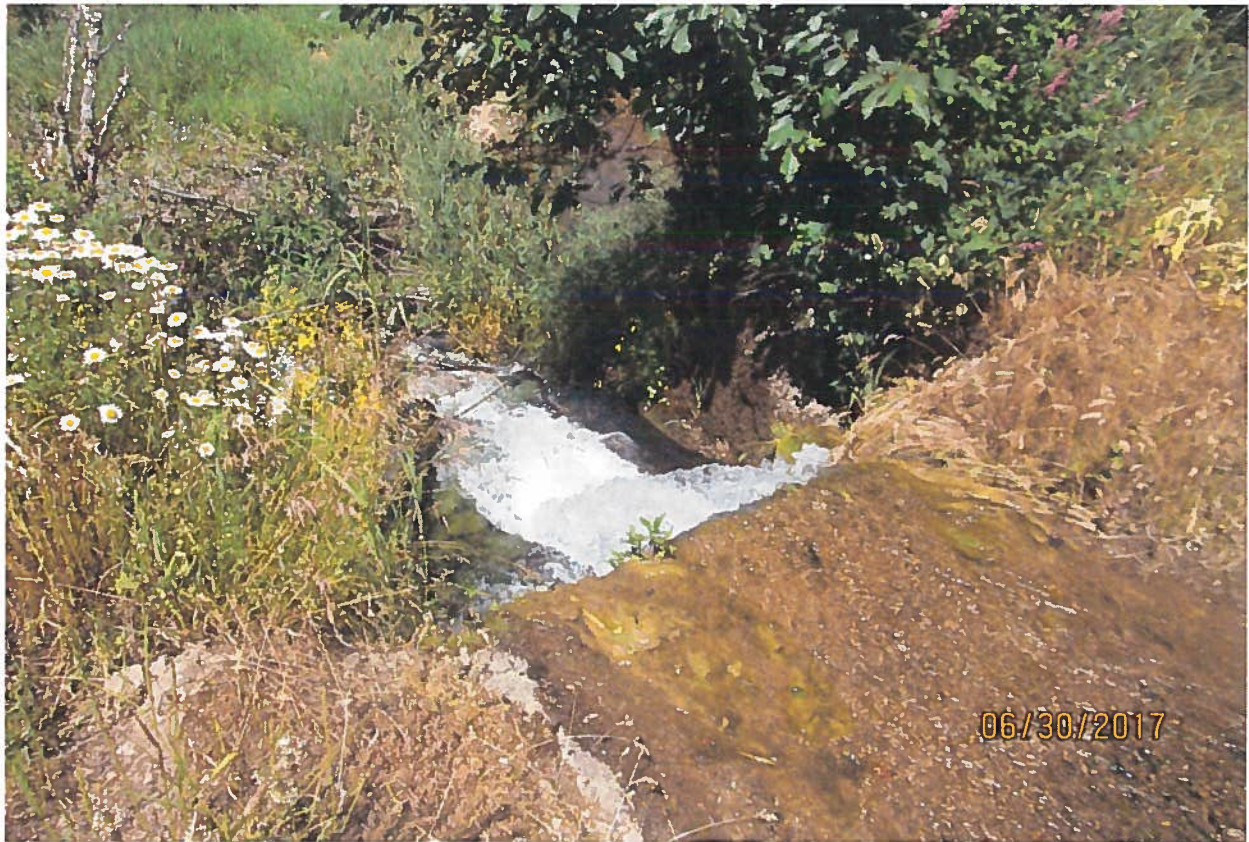
View looking down the 2 nd overflow from pond 3 into Bear Creek.
