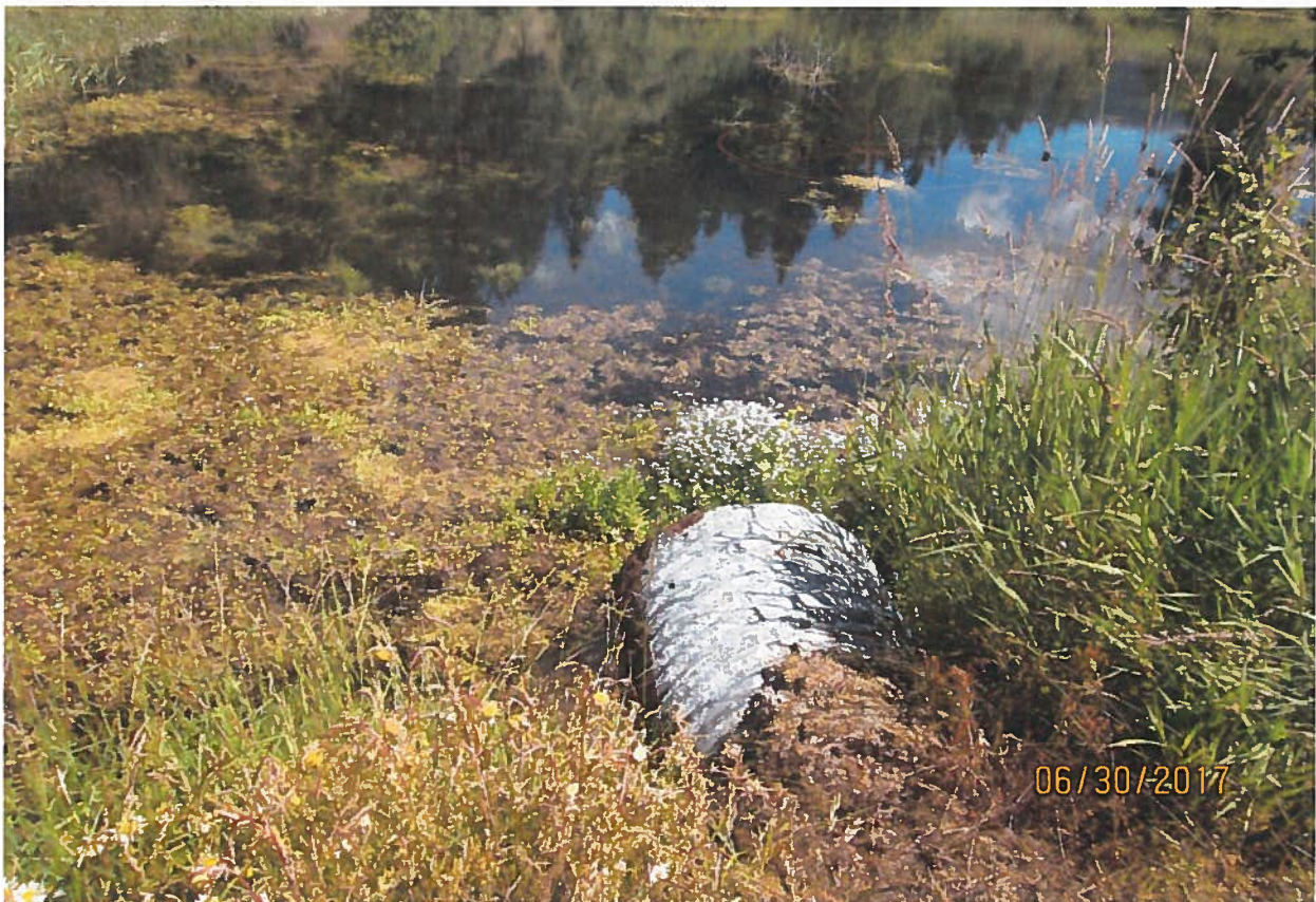
Overflow culvert in between pond 2 & 3. View is looking at pond 2.
