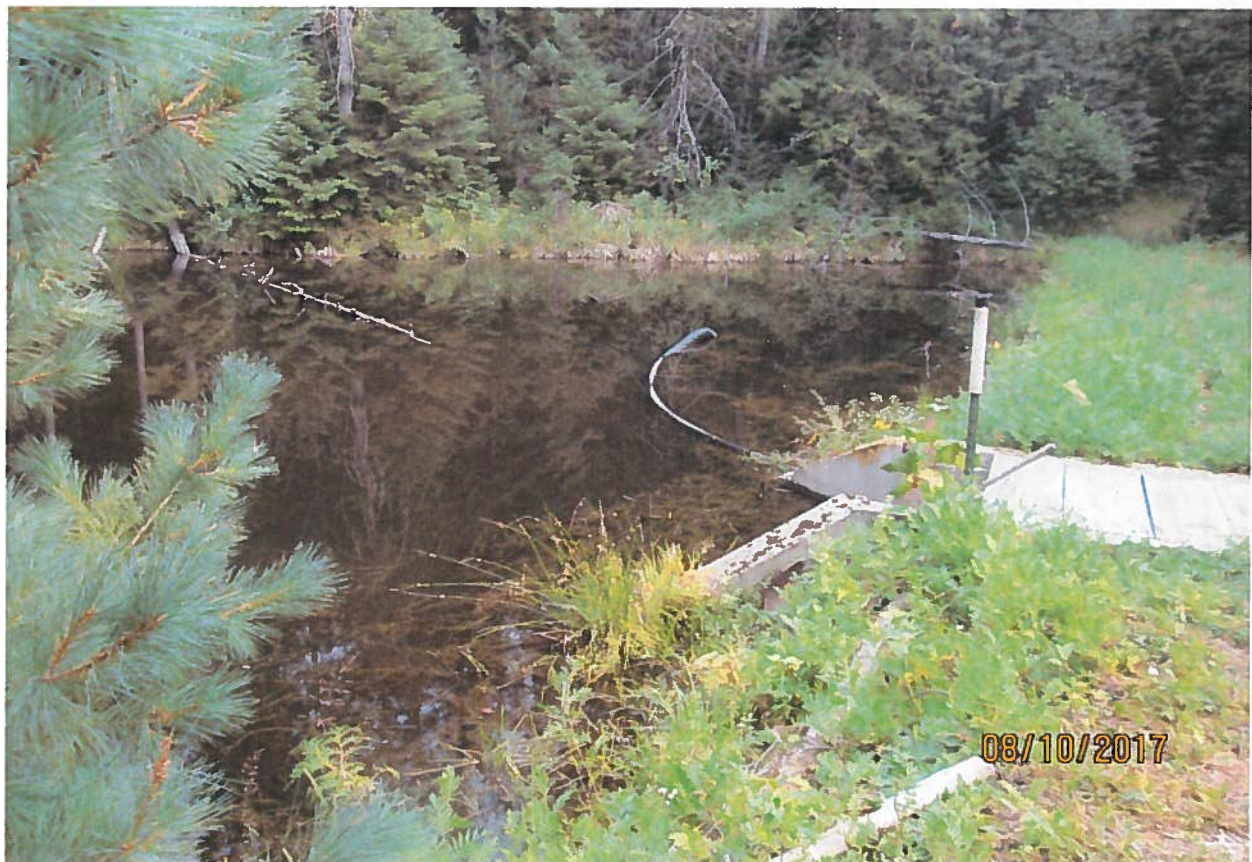
View of storage and dam with outlet structure with bridge over it.
