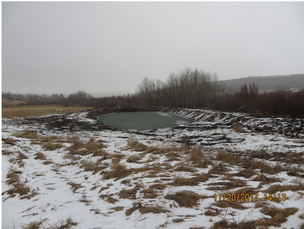
Photo 1a: Pond overview facing in a generally northeast direction.
