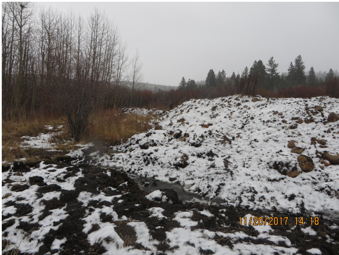
Photo 6: Downstream slope of the main embankment (north end), facing east.
