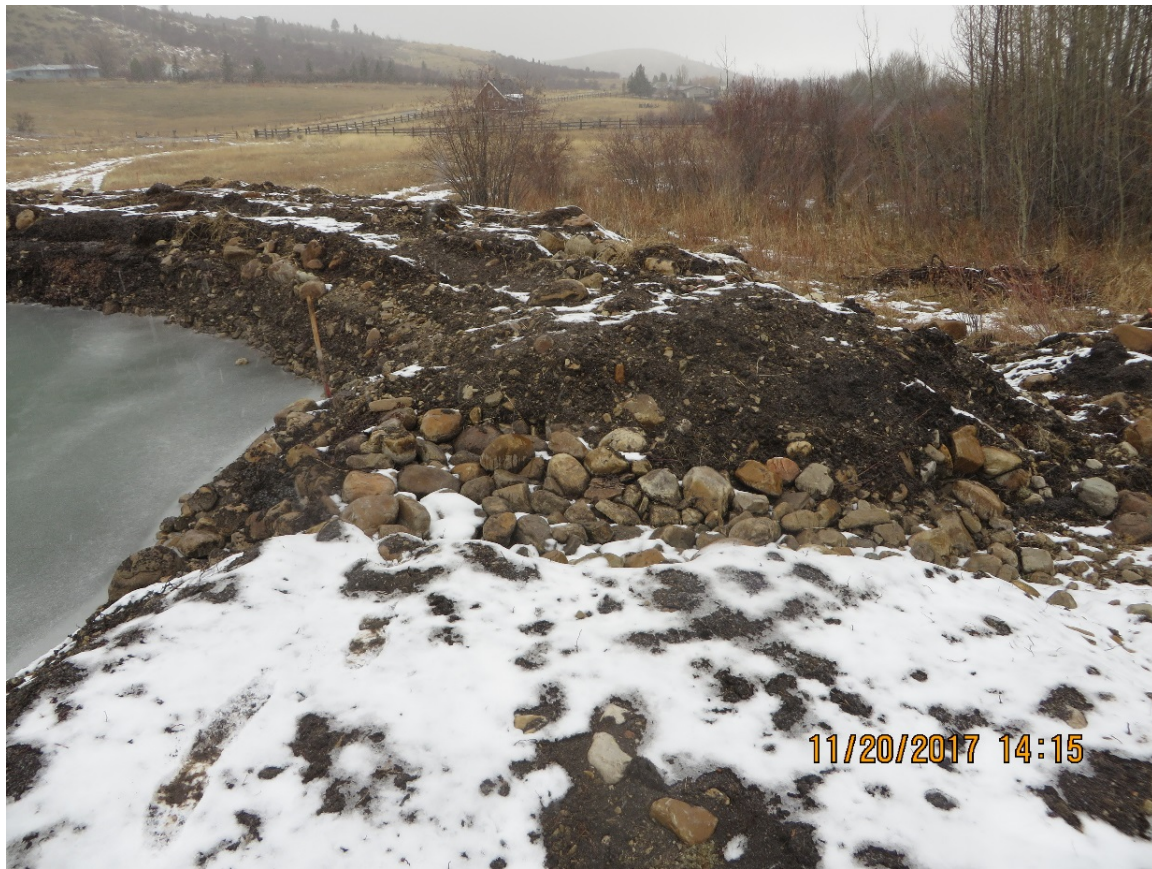
Photo 2a: Spillway channel towards the northeast end of the reservoir.
