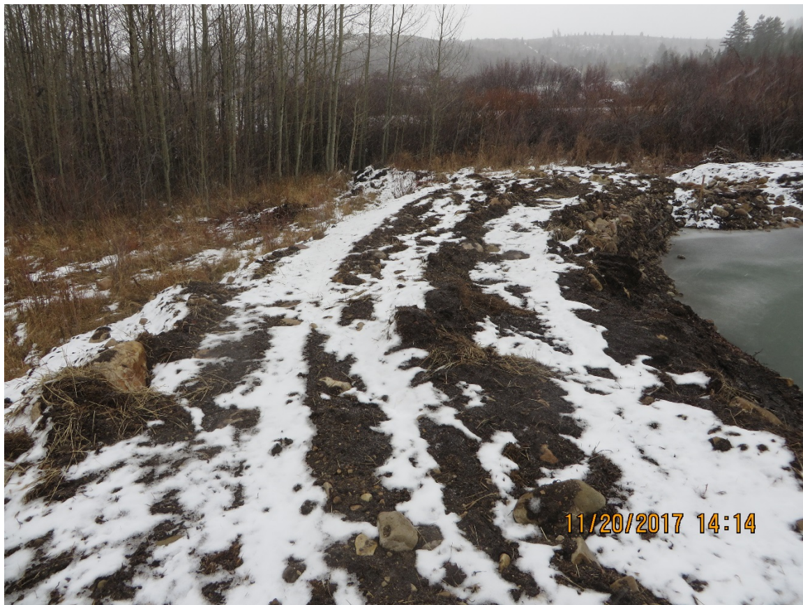
Photo 5: Typical view of the dam crest.
