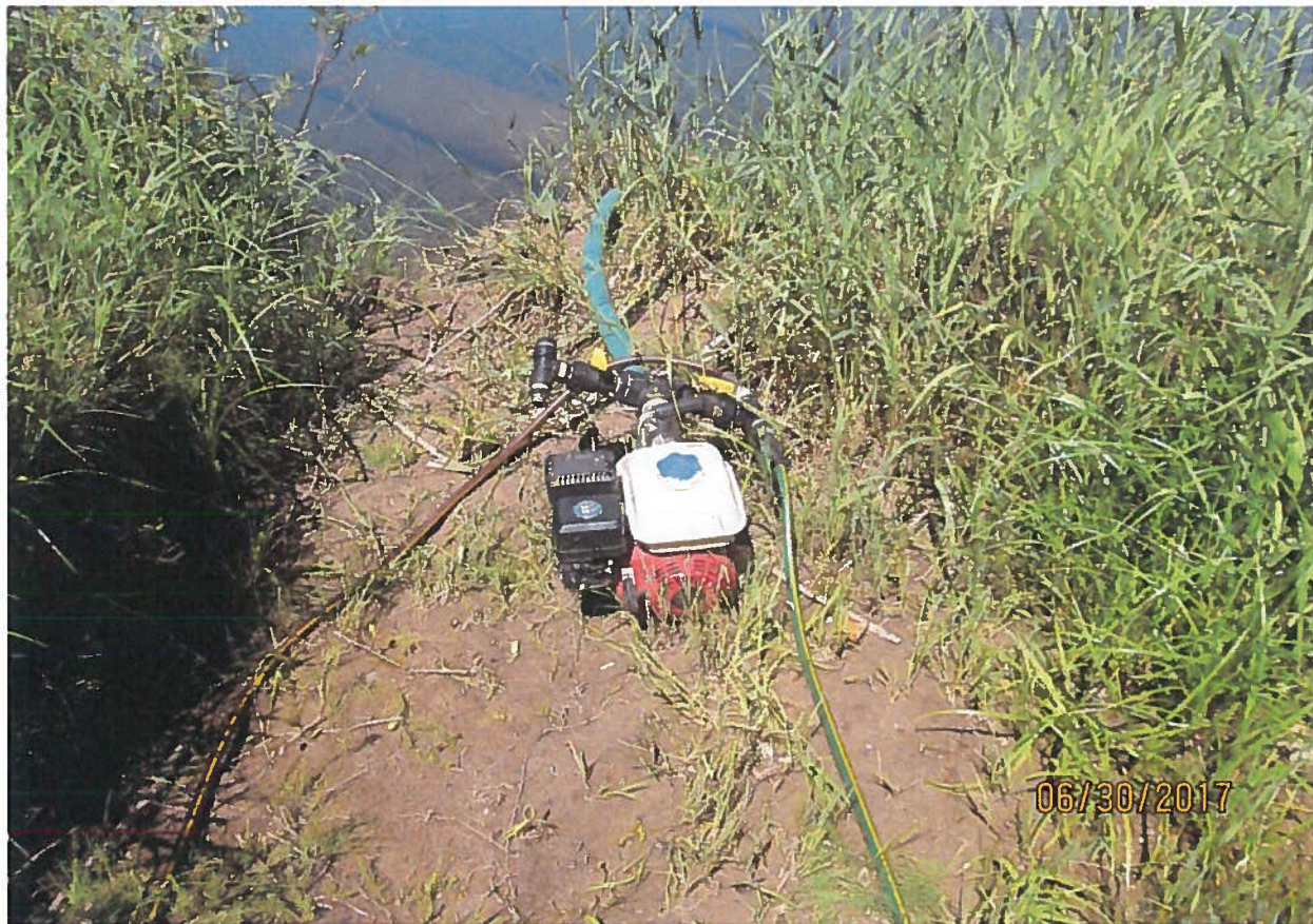
Point of diversion with small portable gas pump.
