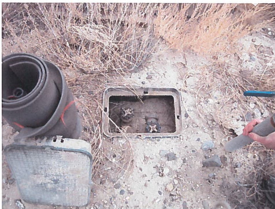
Each of the six greenhouses has a valve for irrigation and one for geothermal heat. The valve on the left is irrigation
