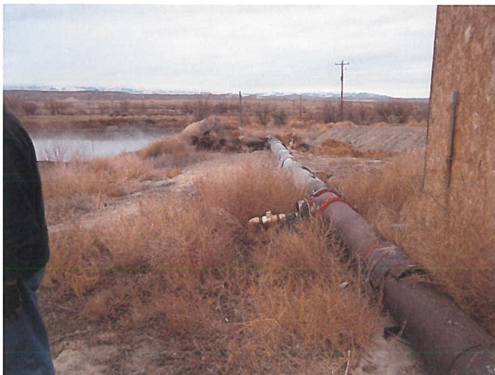
The artesian well provides enough pressure for water to flow up toward the shed. A smaller pipe diverts water to the upper pond for irrigation
