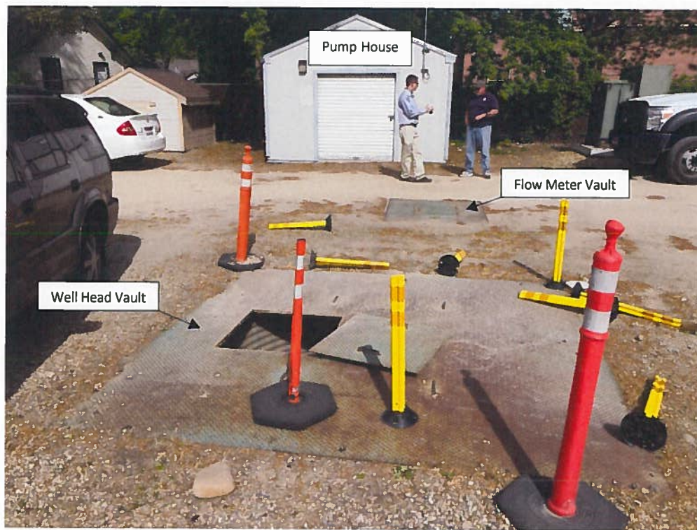
Injection well site
