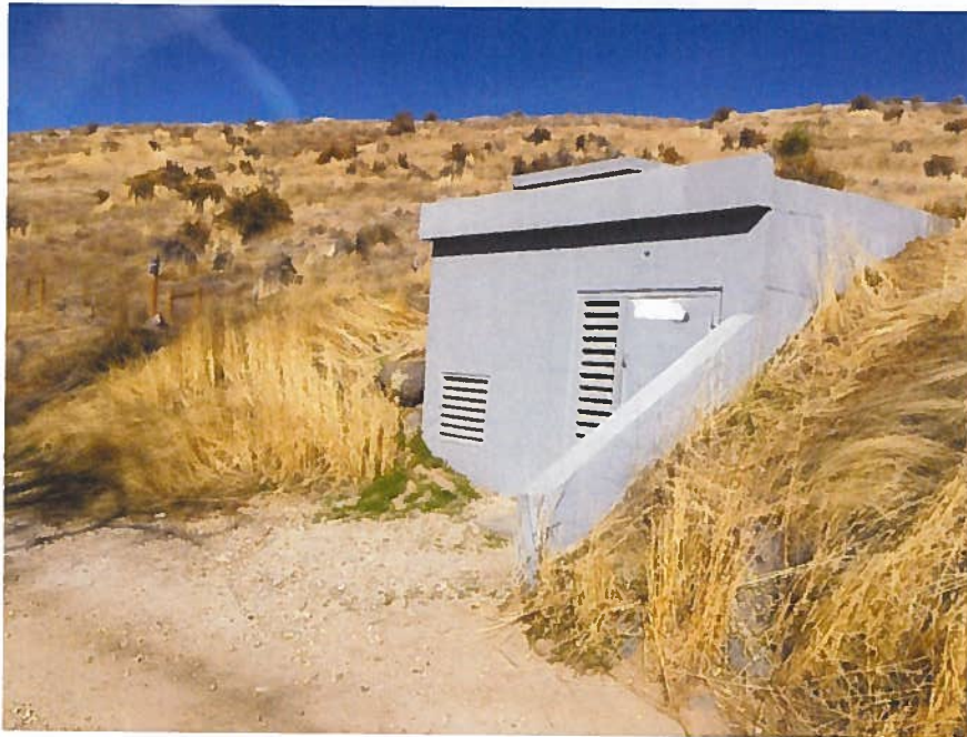
Production Well 4 well house
