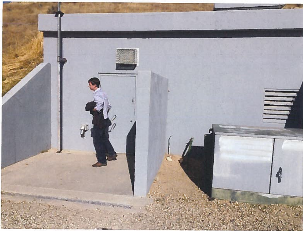
Well 2 well house
