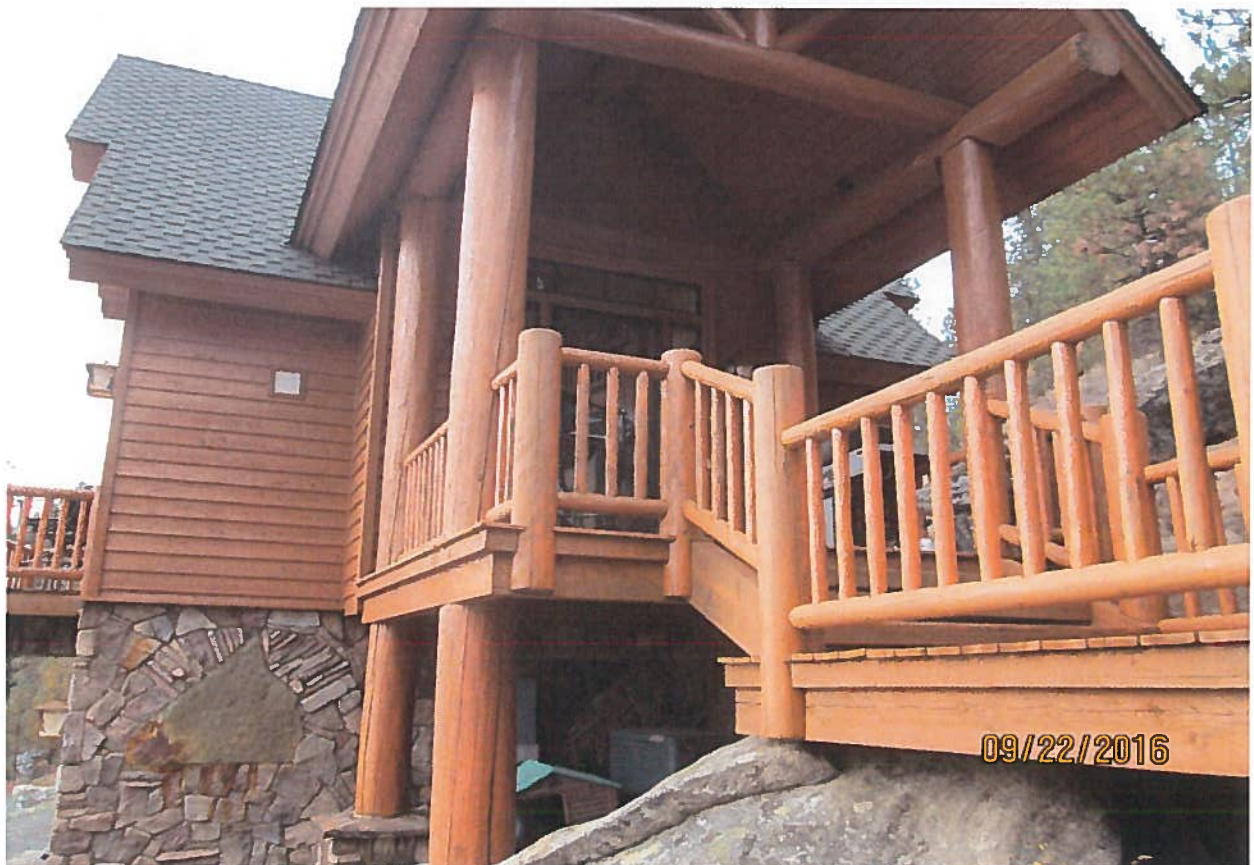
Only 1 home had been built and was using water from the lake.
