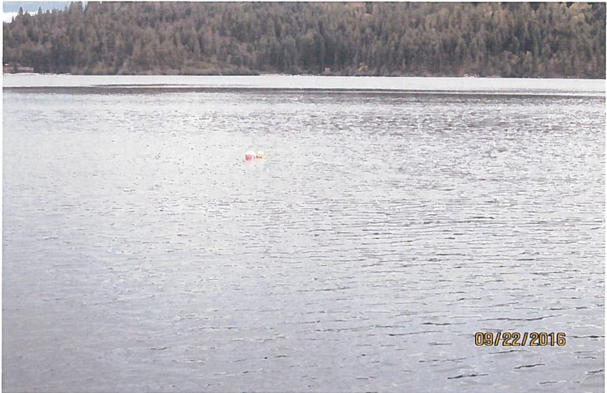
Buoys marking location of pump.
