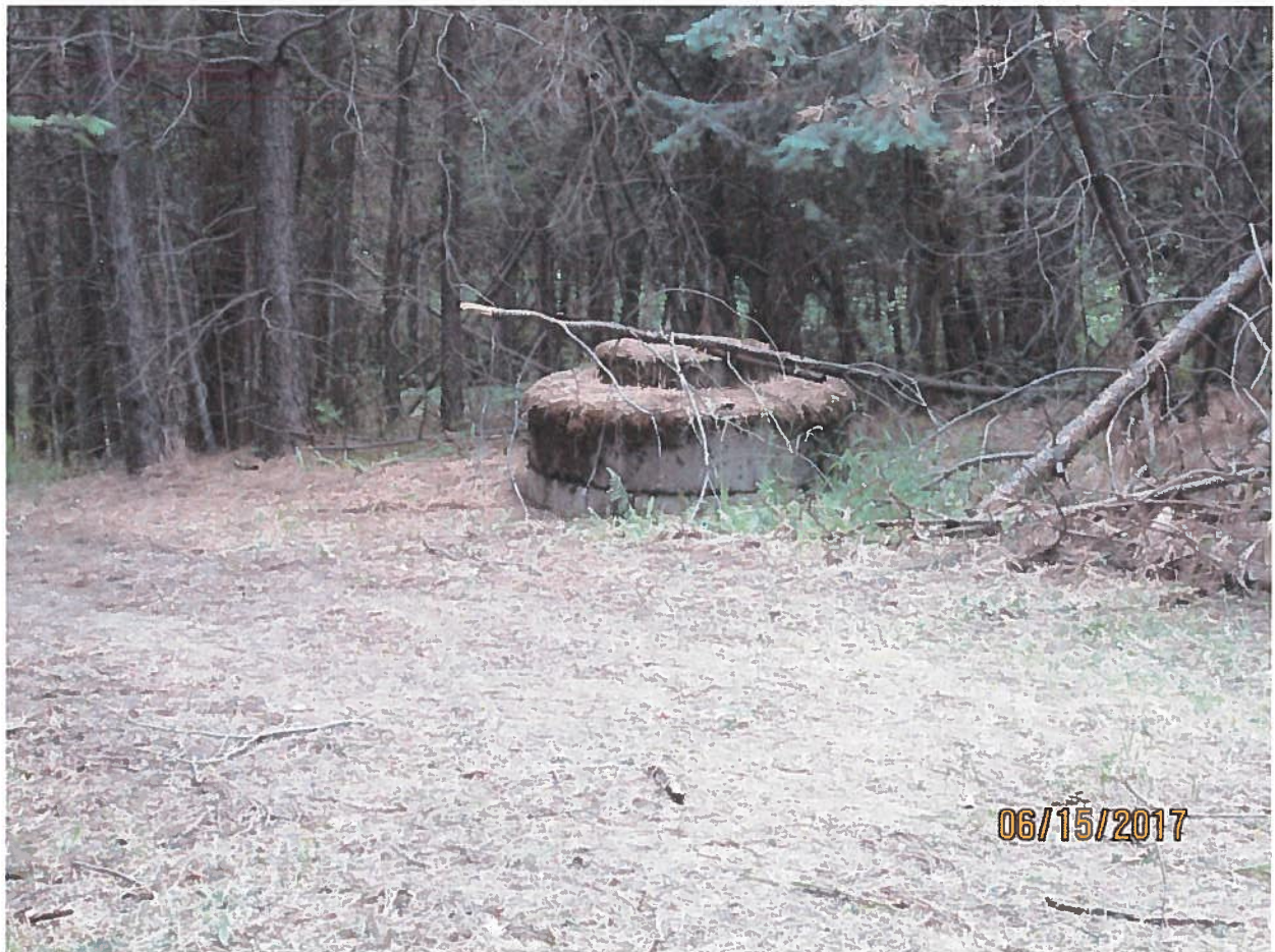
Storage tank 3, also holds 1,500 gallons.
