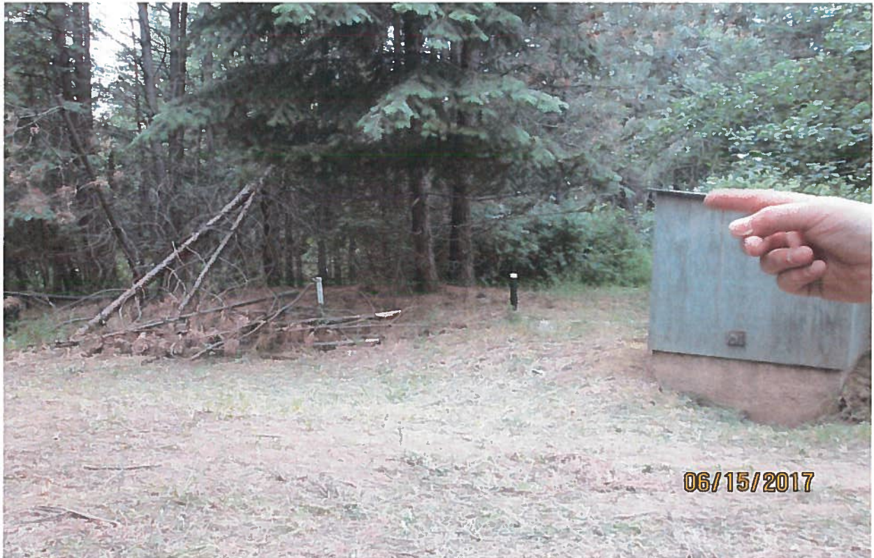
Storage tanks 1 and 2. Each 1,500 gallons.
