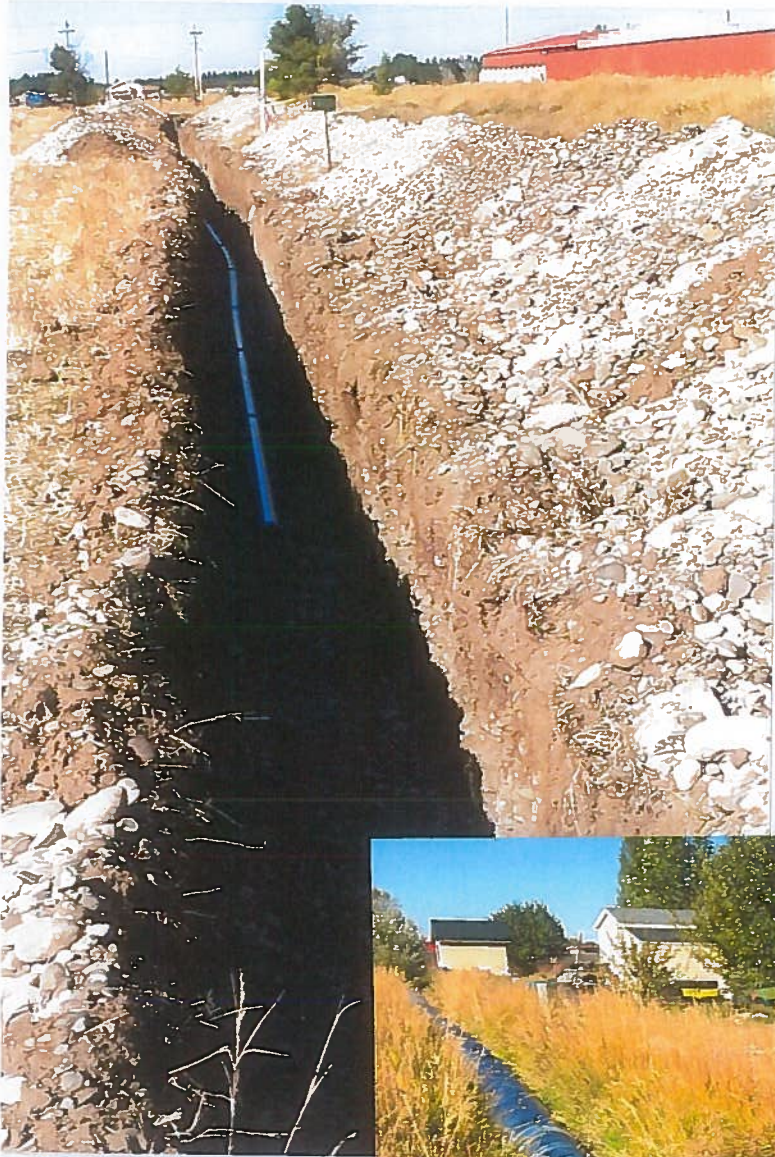
main water pipe for new extension
