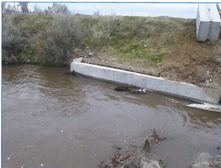
Figure 2: Upper diversion abutment in Canyon Creek and culvert entrance.
