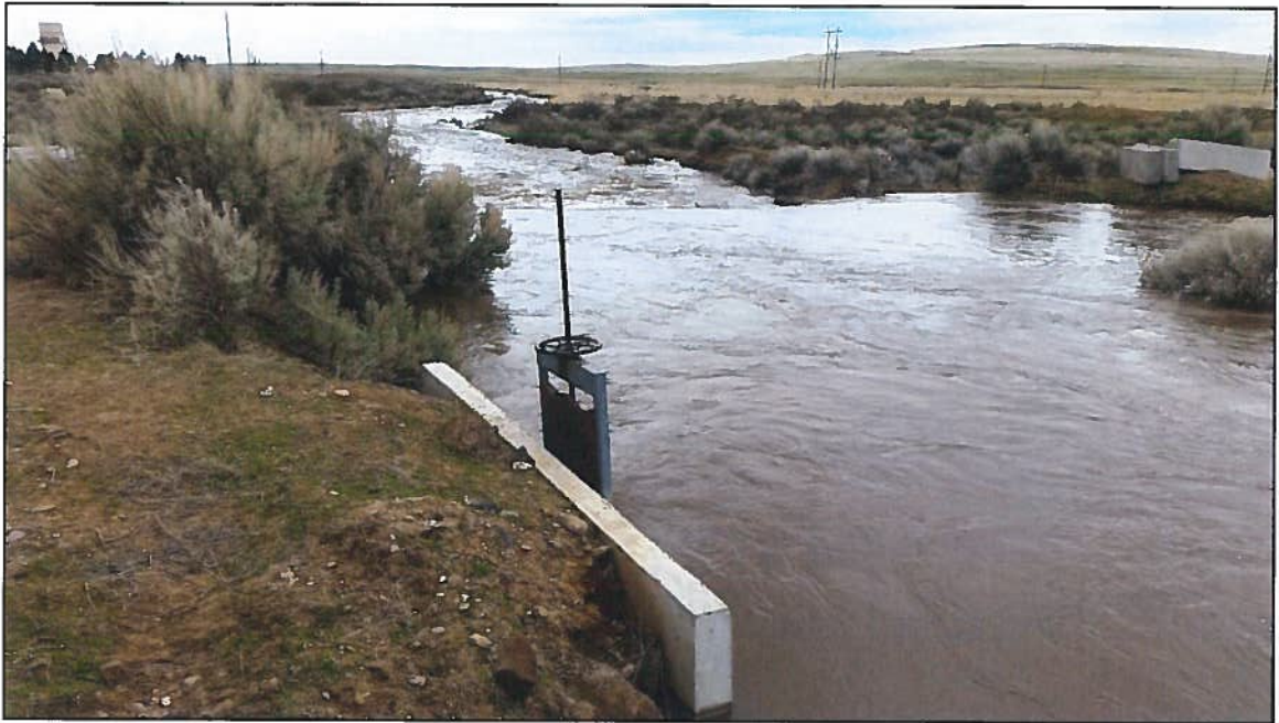
Figure 5: "Lower" diversion headgate from Canyon Creek with check structure in background.
