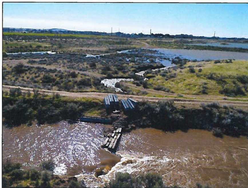
Figure 1: Check structure in Canyon Creek at #1 "Upper" diversion. Just upstream of the check is a concrete abutment on left bank with diversion to the ditch conveying water to recharge areas.
