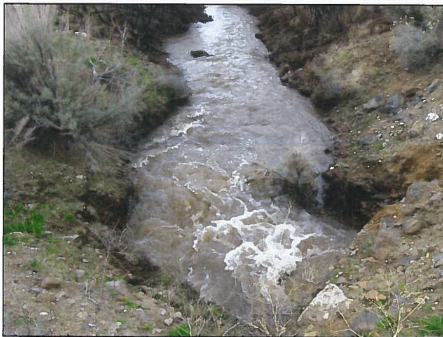
Figure 6: Lower diversion culvert discharge into ditch.
