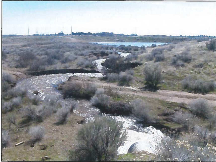
Figure 3: Upper diversion culvert discharging to ditch conveying water to recharge area.
