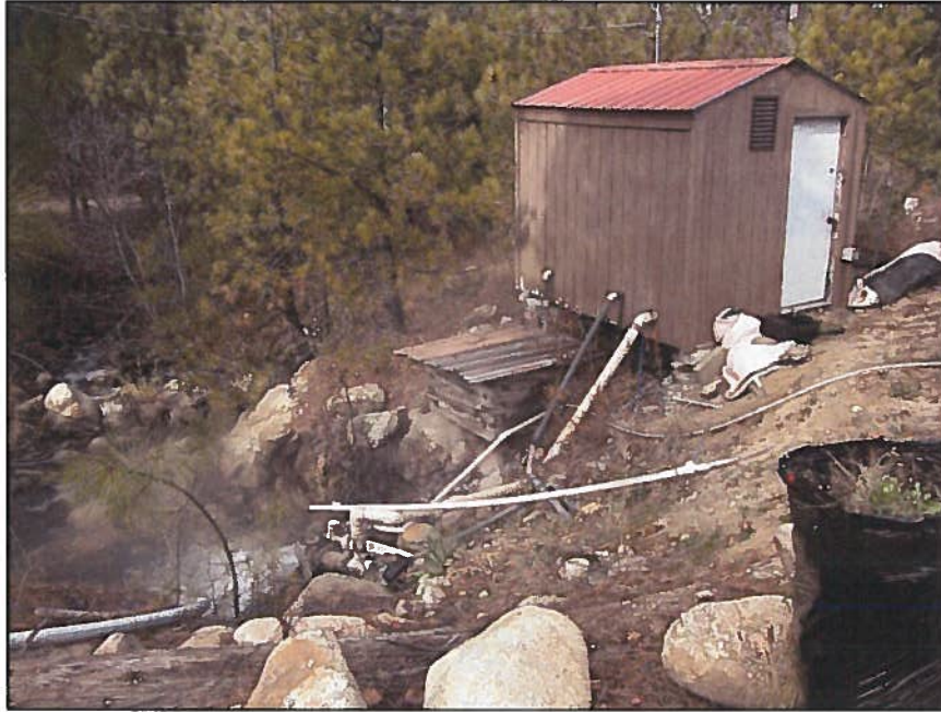
Figure 1: Lower spring pump house. Flow measured at discharge to creek.
