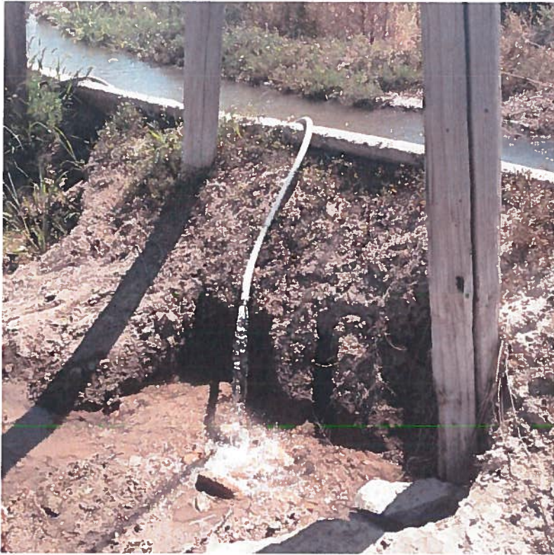
Figure 3 1" siphon tubes draw water from the concrete channels for irrigation.
