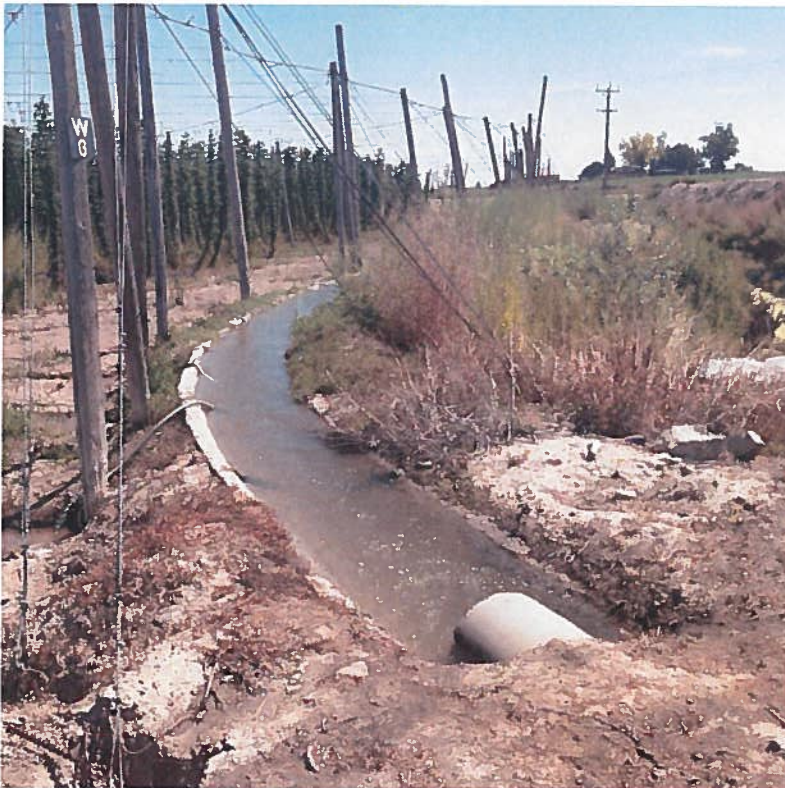
Figure 2 Concrete channels run to the east and west from the well to convey diverted water to the POUs for both rights
