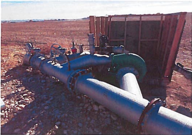
Pressure Reading at 2nd Booster Pump
