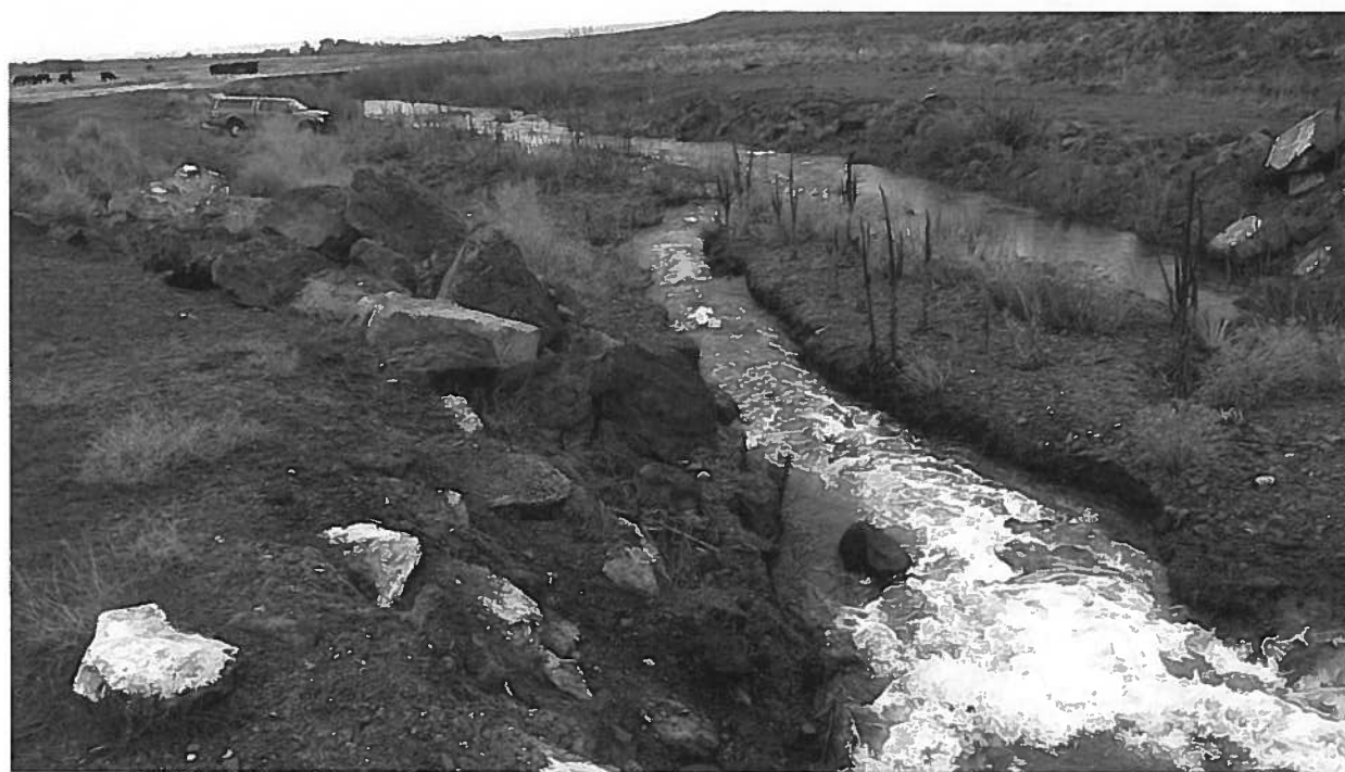
Photo 5. Looking downstream Canyon Creek from diversion structure.
