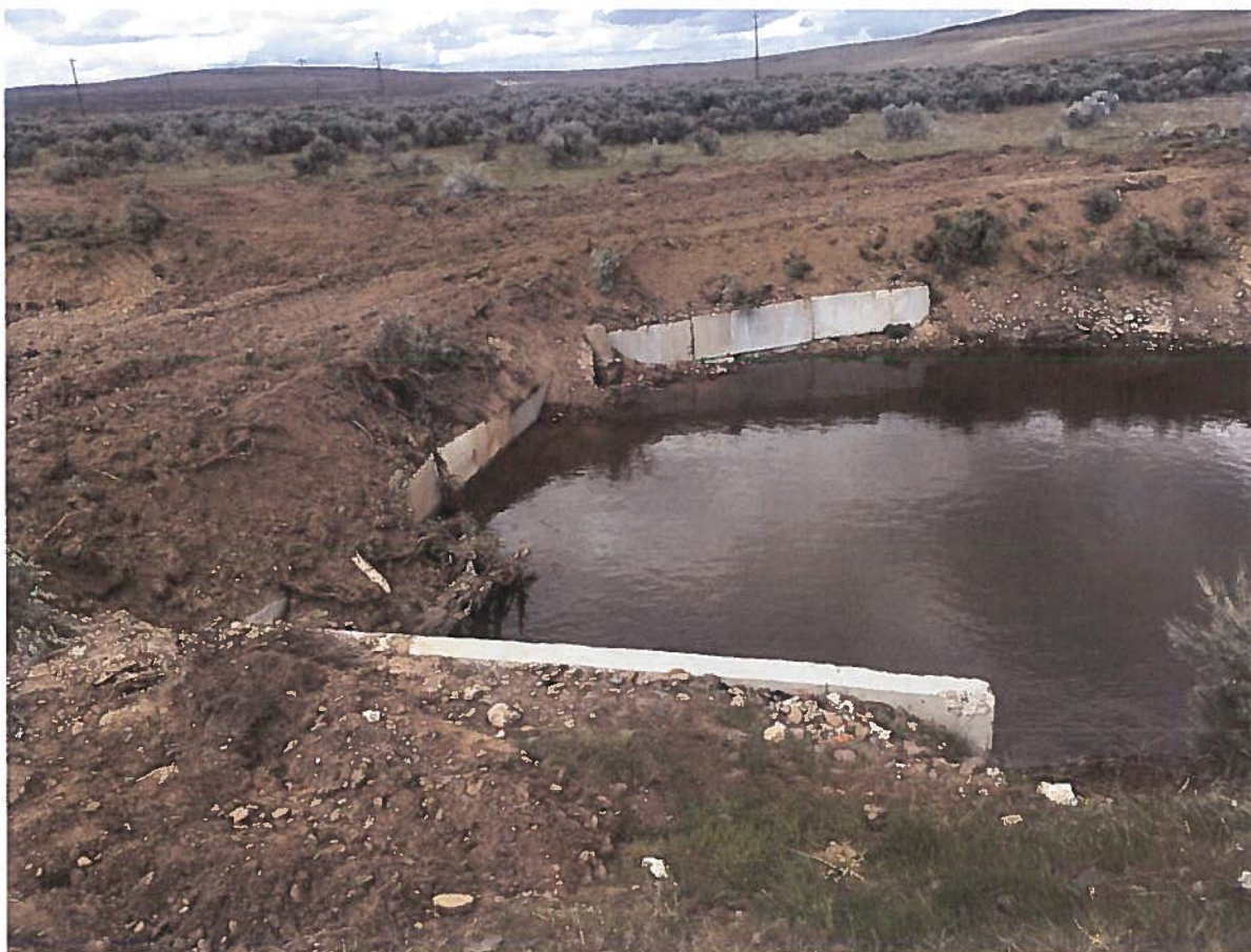
Photo 6. Check dam at Canyon Creek diversion structure. Photo taken on 4/20/2017
