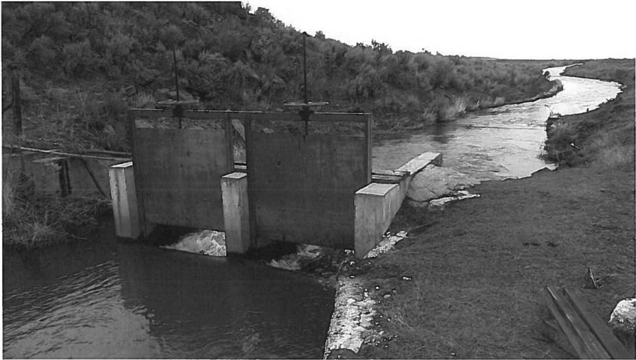
Photo 2. Headgate structure on the Mountain Home Canal.
