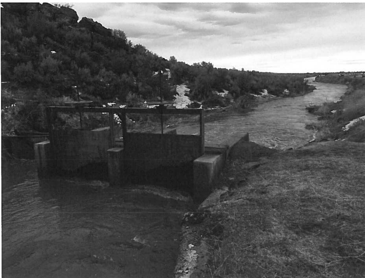
Photo 2. Head gate structure on the Mountain Home Canal. Photo taken on 2/9/2017.
