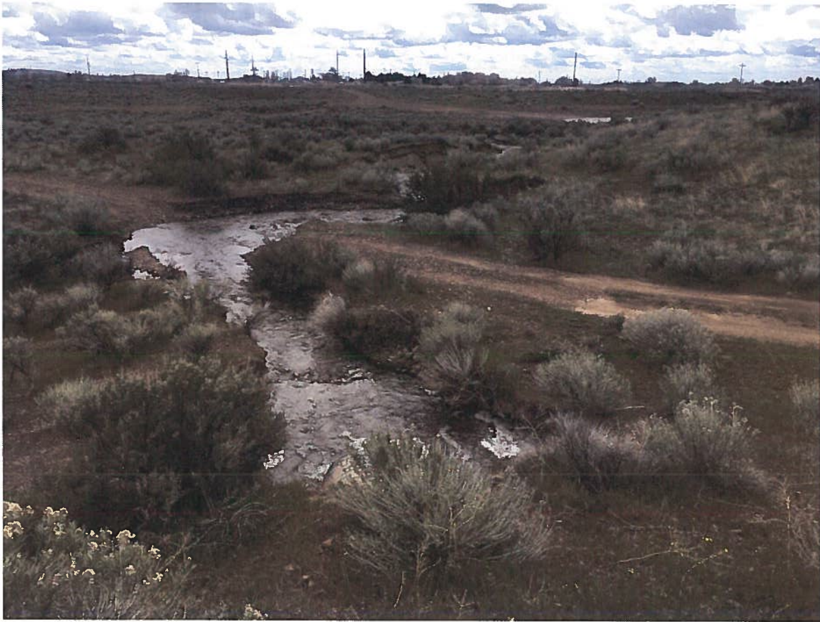
Photo 4. Diversion into gravel pit. Photo taken on 4/20/2017.
