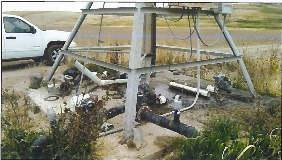
Figure 4: Interconnection between Well 1 and Well 2 occurs at the mini pivot in Section 20 NWNENW.
