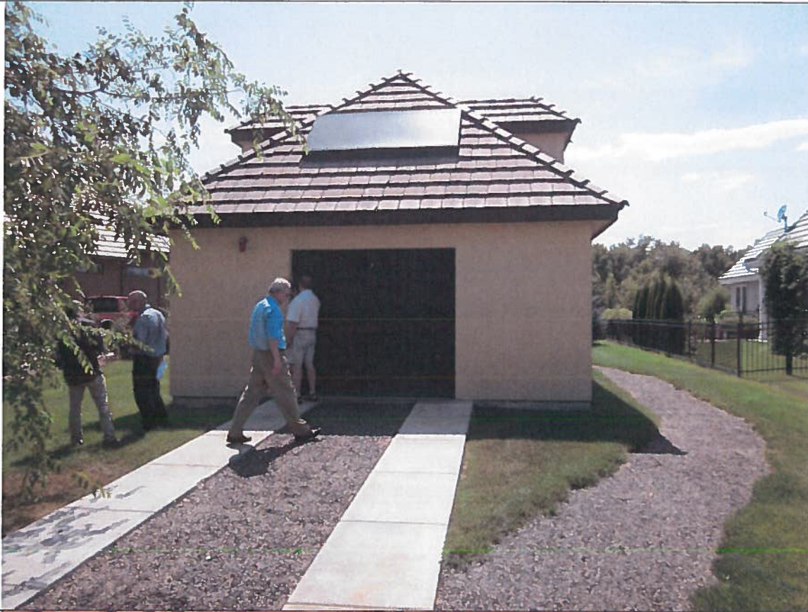
Pump station on the south side of the round a bout on W. Sherington Court.
