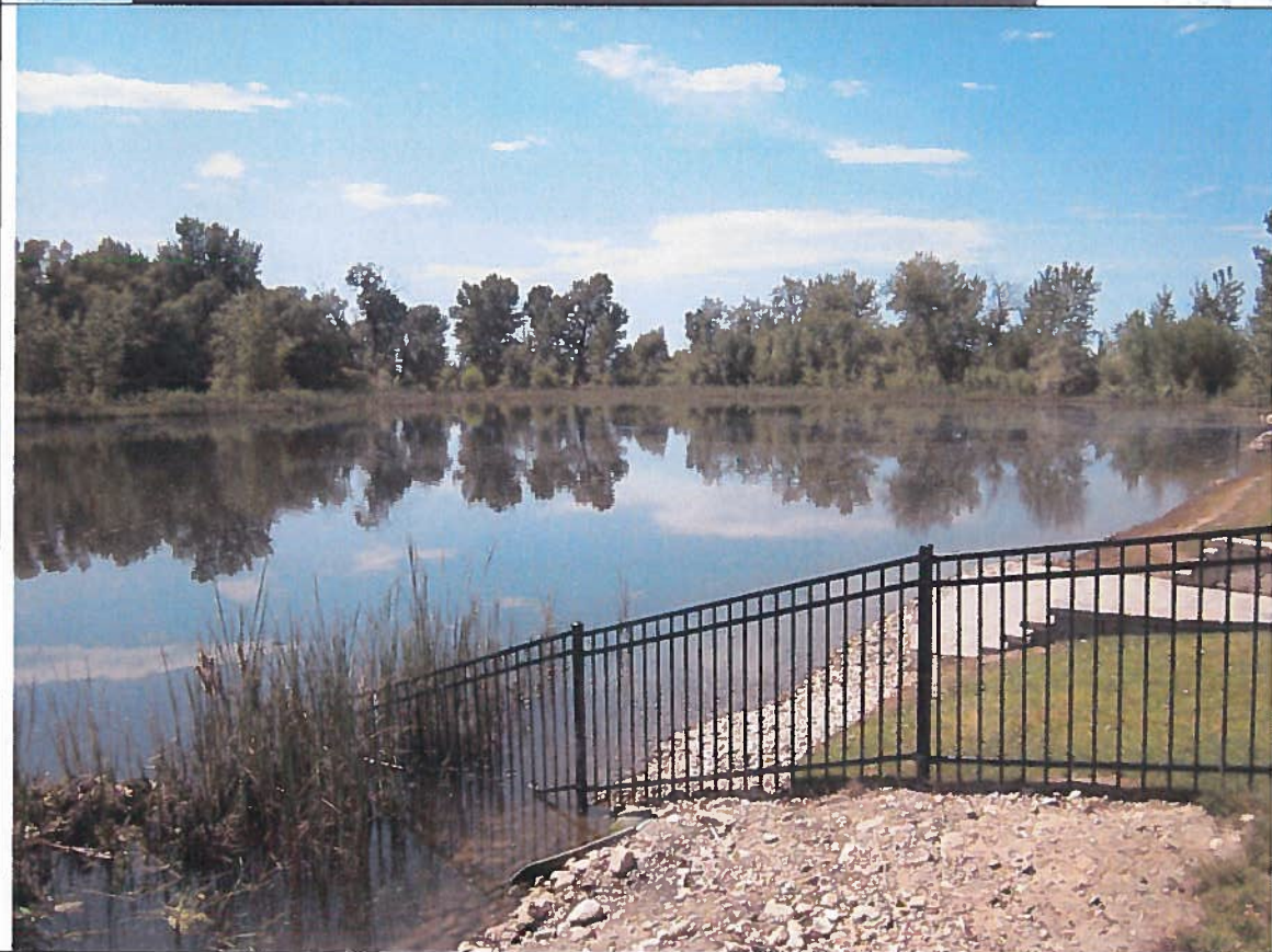
Pond 4 looking southwest. The water is about 4 feet higher than what is normally is due to the high water year. This is a common area behind the pump station.
