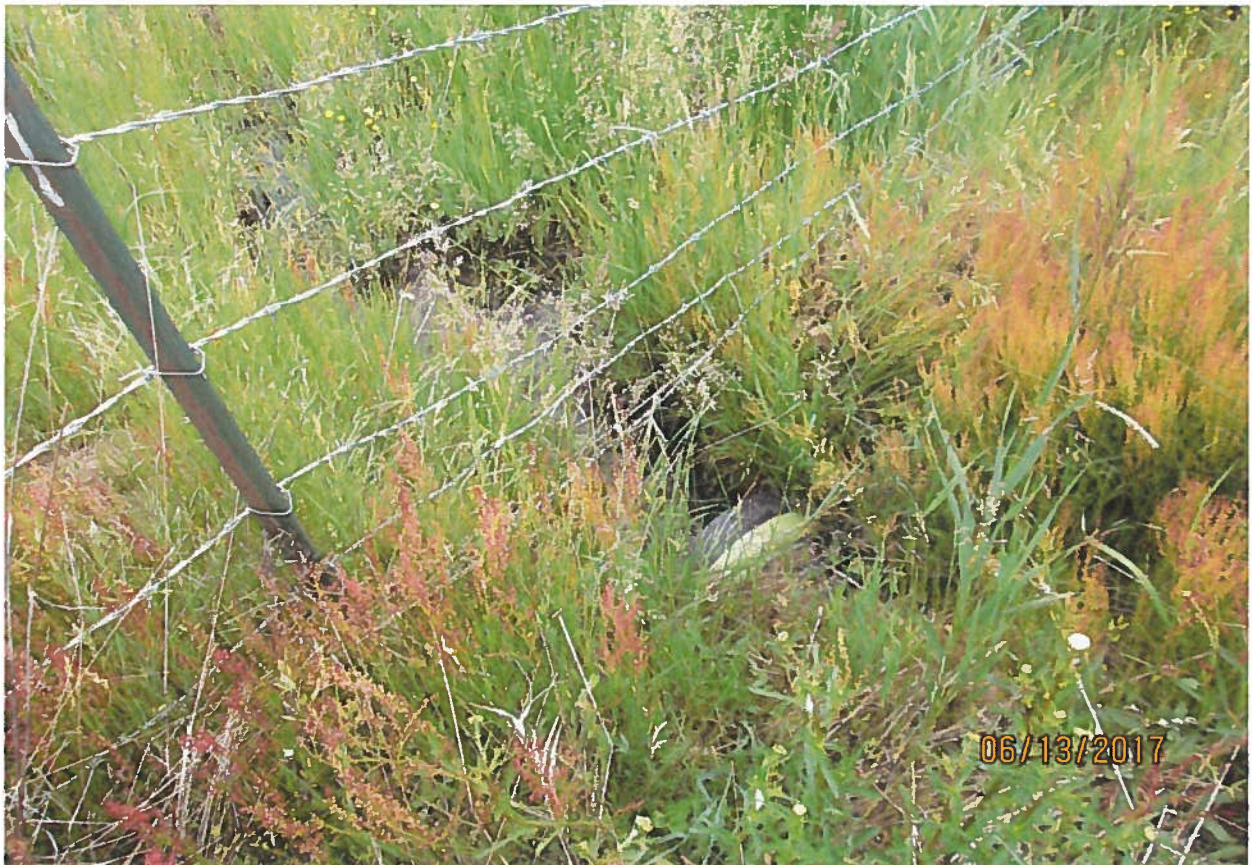
Culvert from pond allowing overflow to Benewah Creek.
