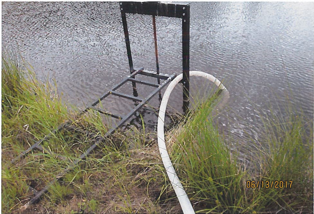
Point of diversion.
