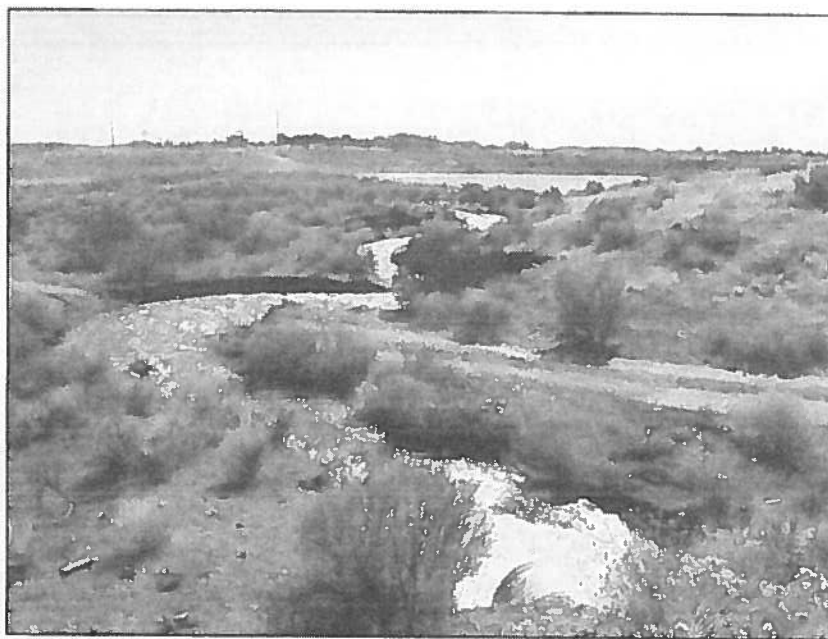
Figure 3: Upper diversion culvert discharging to ditch conveying water to recharge area.
