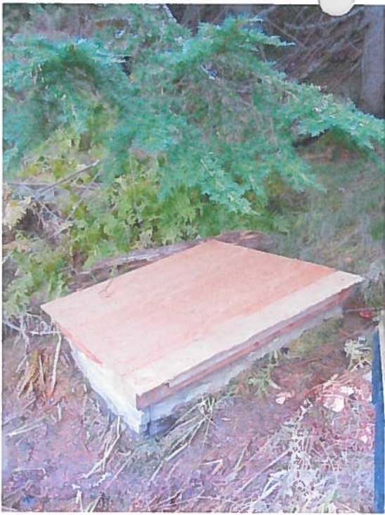
Redwood springbox wit 1/2 Hp pump Located above beaver pond that drains into Grouse Creek
