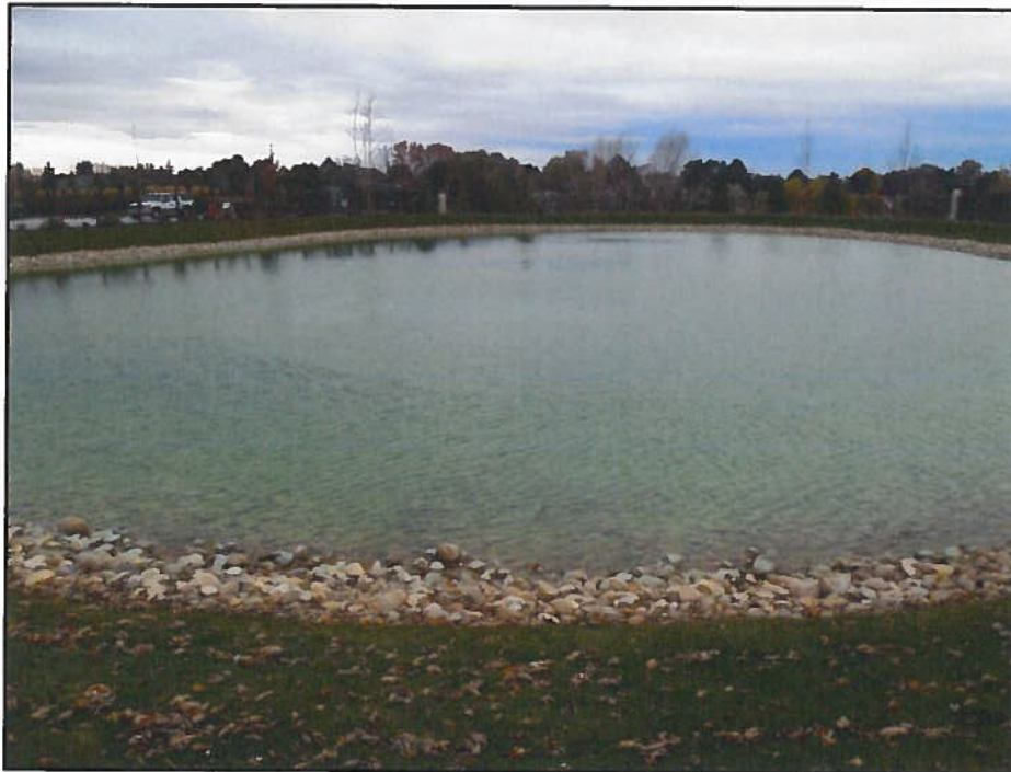
Figure 6. Lower pond (looking west)
