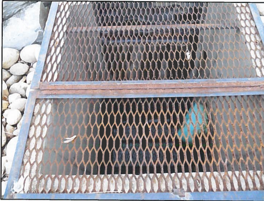
Figure 7. Weir (south side of upper pond)
