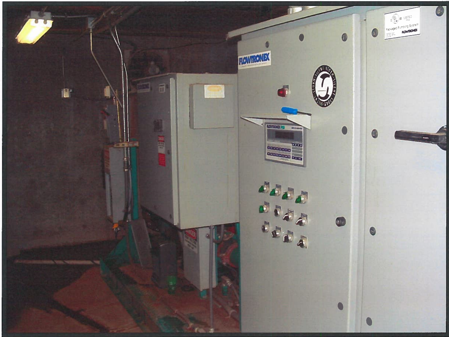
Flowtronex Pump System at Whitetail Pond
