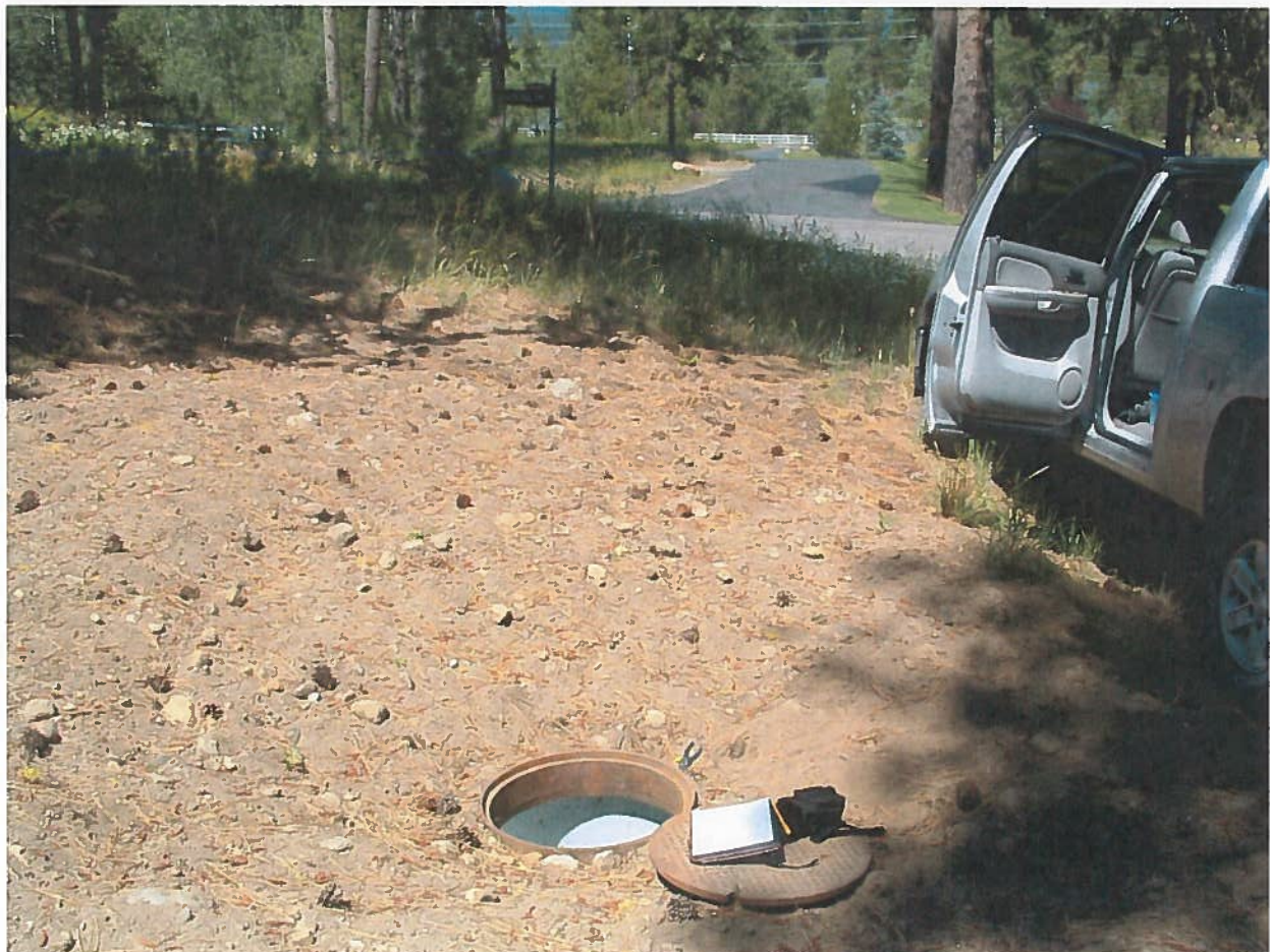
Figure 2 – Flow meter manhole looking north. Intersection of Whitetail Drive and the maintenance shop access is in the background
