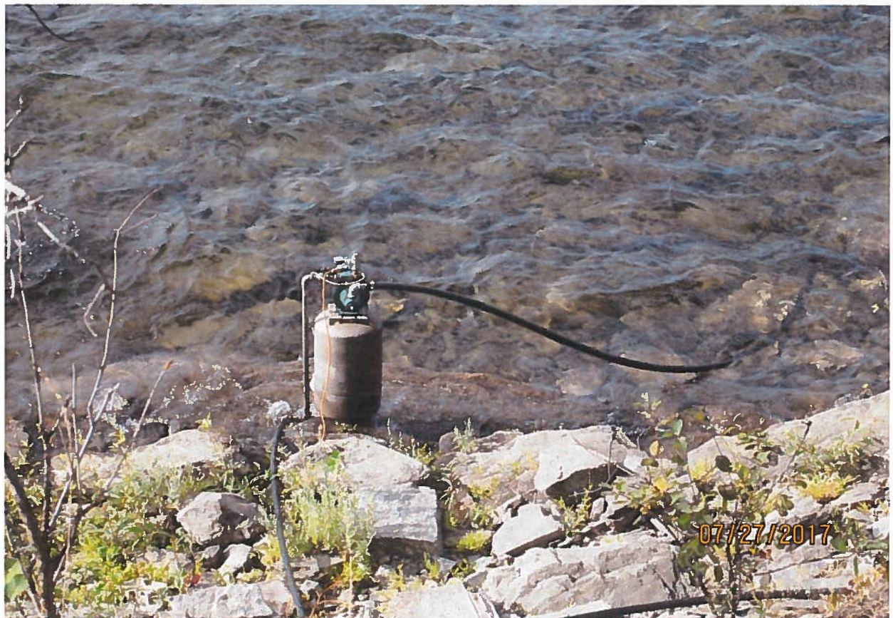
1 inch pipe going into lake. 1hp pump with pressure tank. Pump produced 20gpm or 0.04 cfs.
